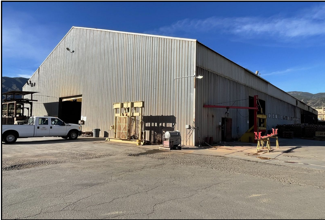
PHOTOGRAPH 1 Building A, Looking Southwest
