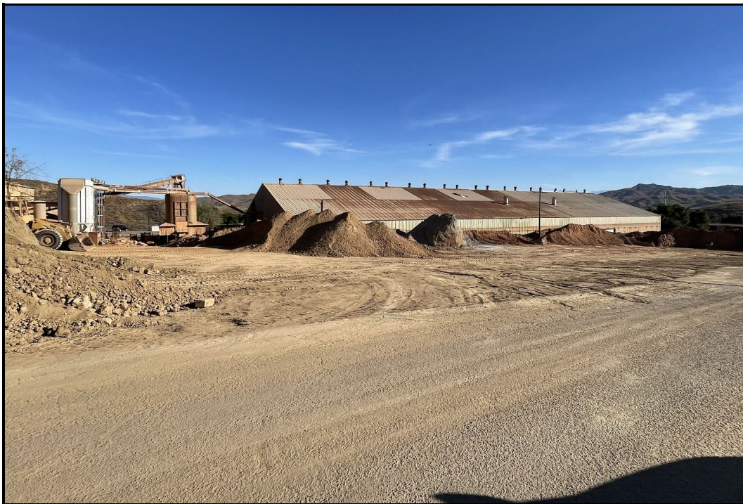
PHOTOGRAPH 4 Backside of Building A with Dirt Piles, Looking Northeast
