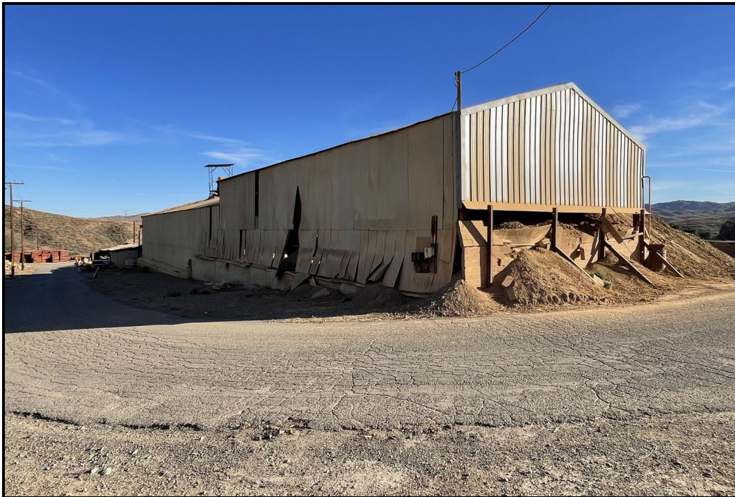
PHOTOGRAPH 2 Buildings B and C, Looking Northeast
