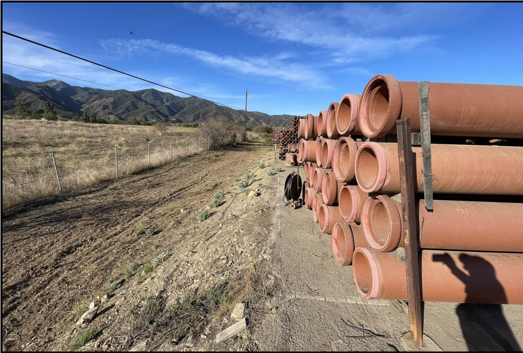
PHOTOGRAPH 8 Elevated Graded Pad along the Southern Boundary, Looking West
