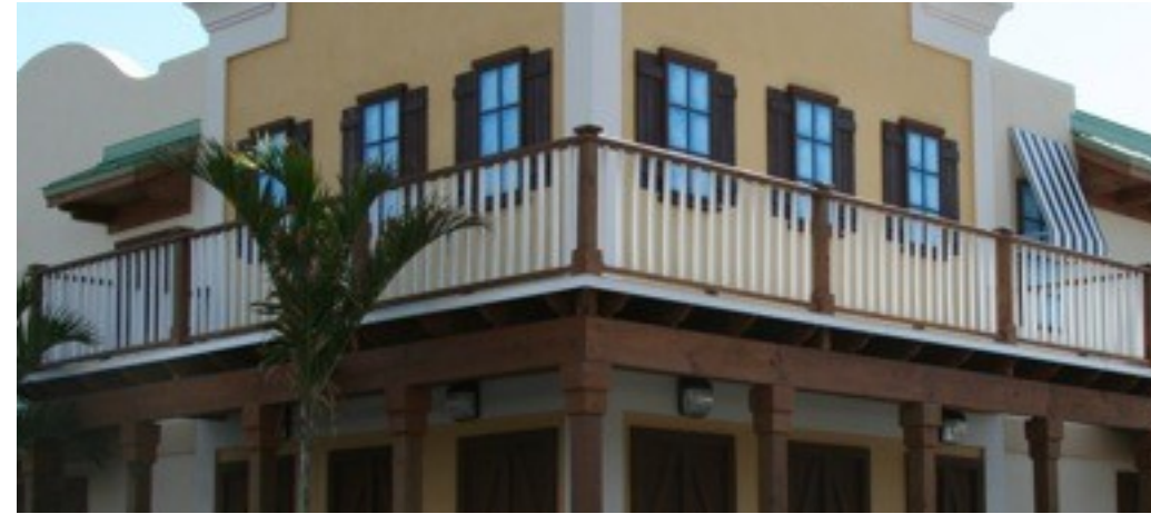
Second Story Elements Real or Faux Windows, Additional Architectural Elements (Rails, Shutters, etc.)
