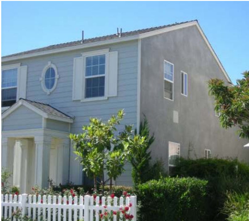
Transition - stucco / siding
