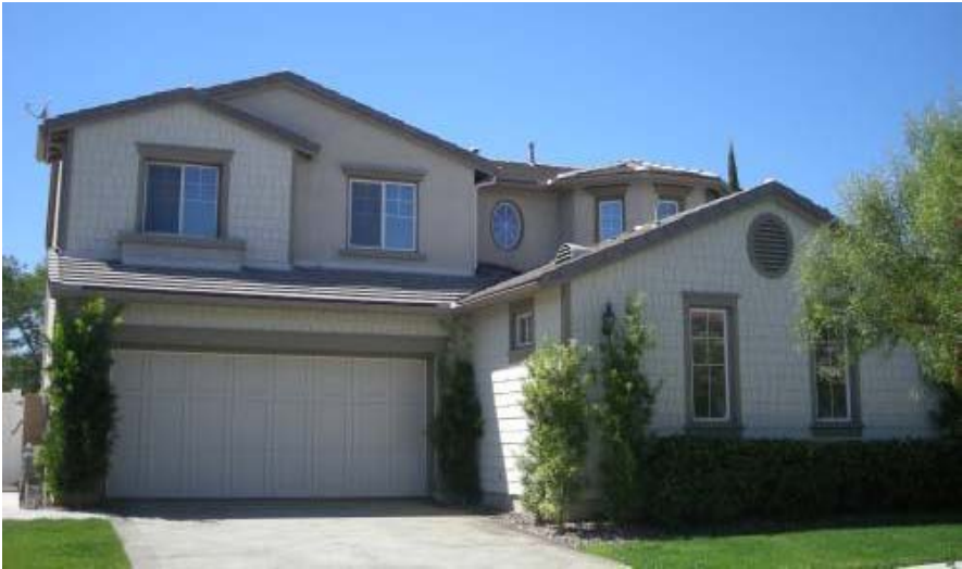
Material Break - siding / stucco
