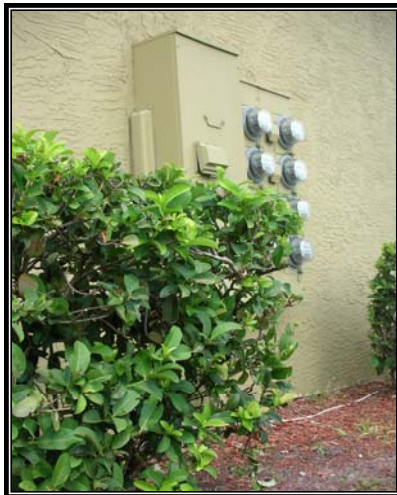
To reduce its visual impact, of wall-mounted equipment may be screened by landscaping or painted the same color as the primary structure.
