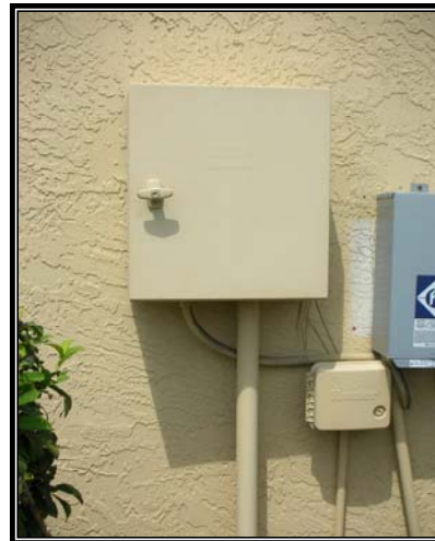
To reduce its visual impact, of wall-mounted equipment may be screened by landscaping or painted the same color as the primary structure.
