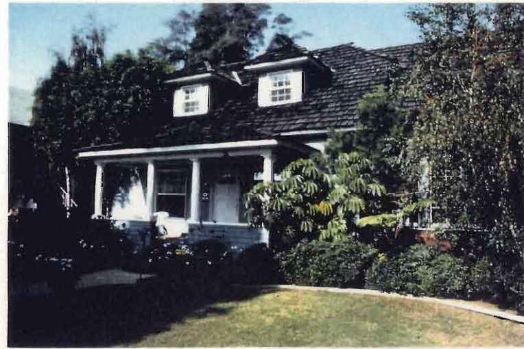
PORCH AND DORMER WINDOWS
