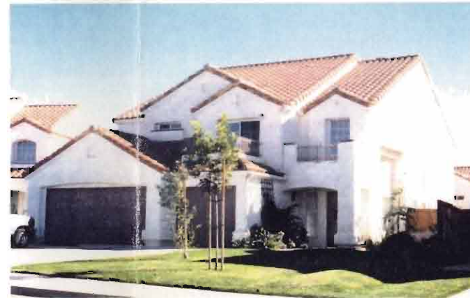
STEPPING GARAGE DOORS
