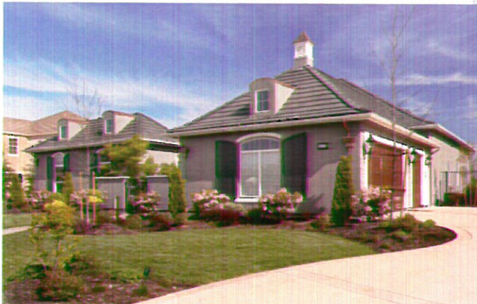
Side-entry allows for an interesting street elevation
