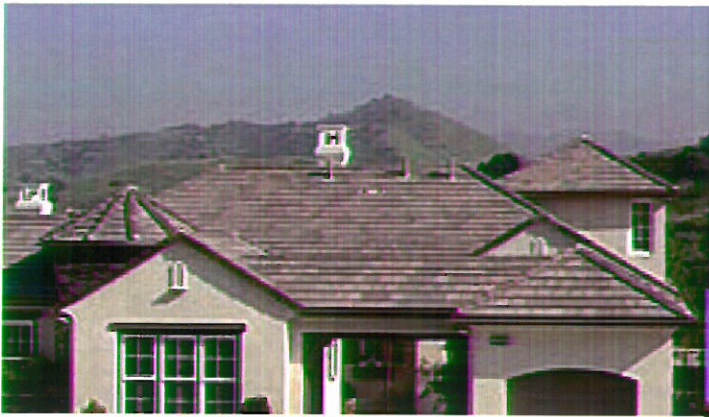
French Country roofs - flat concrete tiles ranging in color from light to dark
