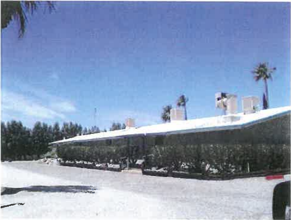
MAIN CLUBHOUSE WITH SWIMMING POOL
