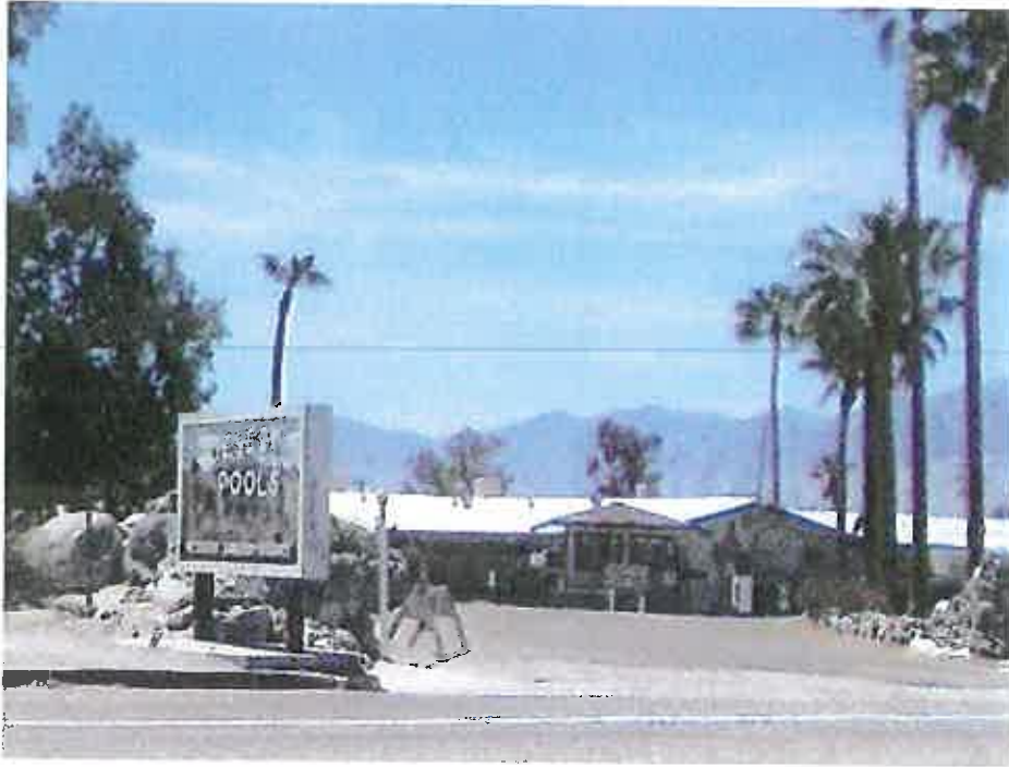
ENTRY CLUBHOUSE STORE AND SWIMMING POOL
