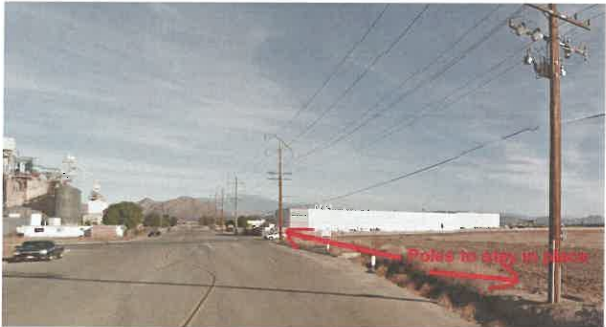
Power poles along Rider Street are just feet from the roadway.
