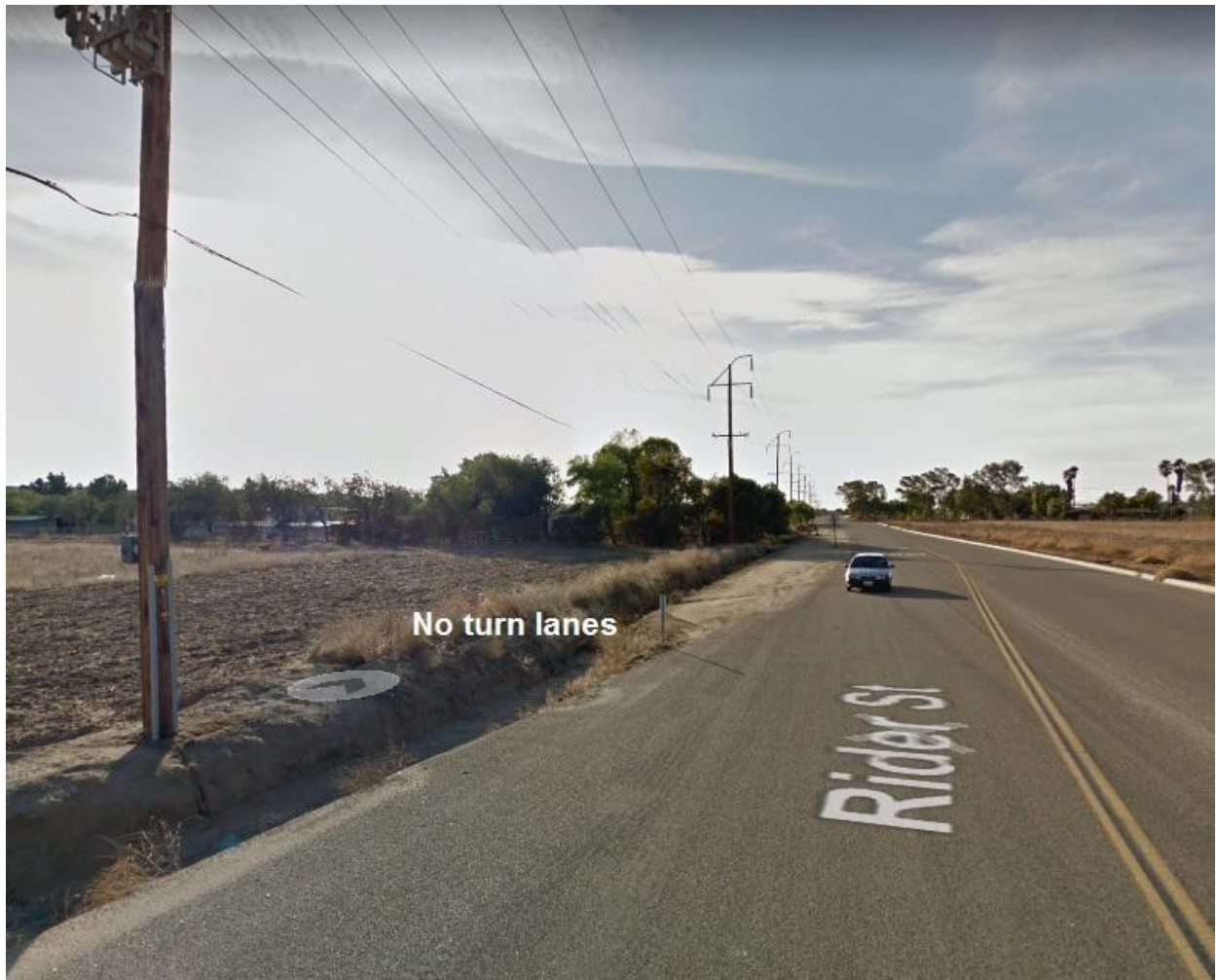
Power poles are just feet from the road.
