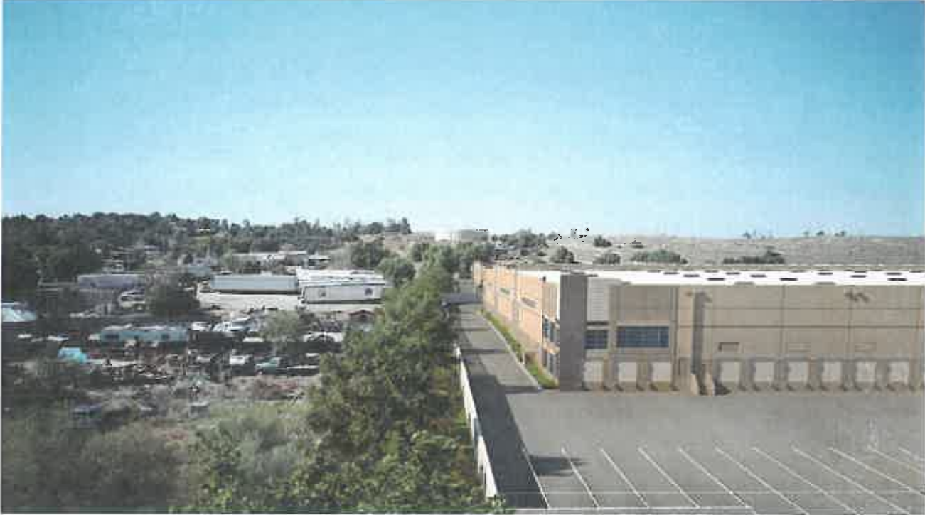
Building D Southern Boundary Viewed from the East
