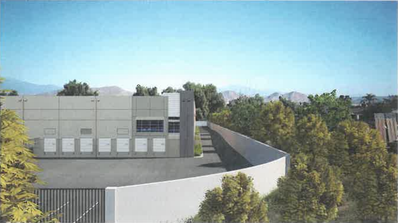
Building D Southern Boundary Viewed from the West
