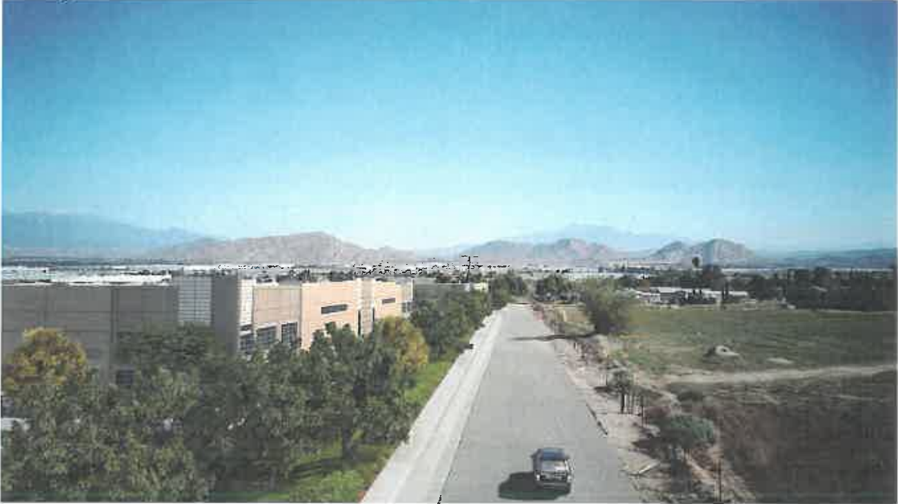
Building E Southern Boundary Viewed from the West
