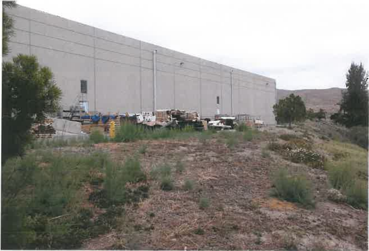
PHOTO # 03: PROJECT AREA #1
