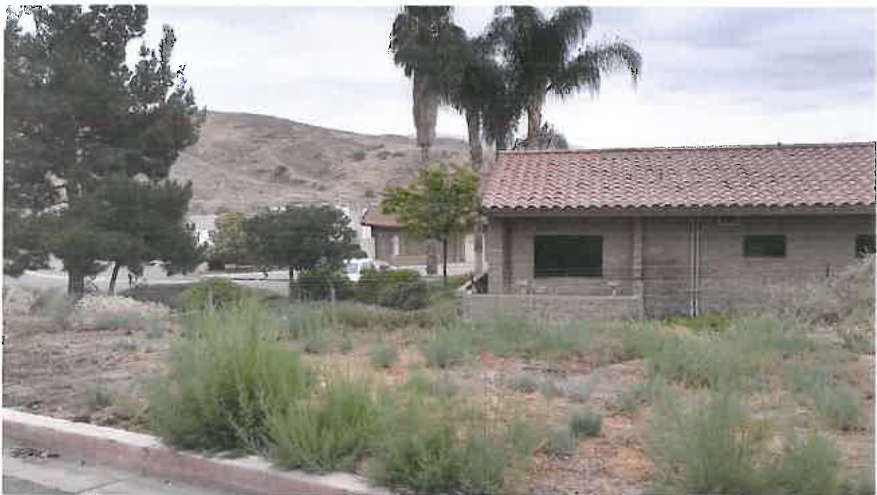
PHOTO # 06: PROJECT AREA #4
