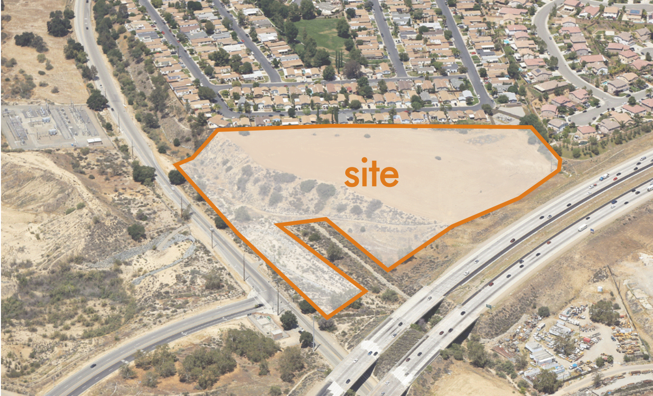
Figure 1-5 Additional Site Views
