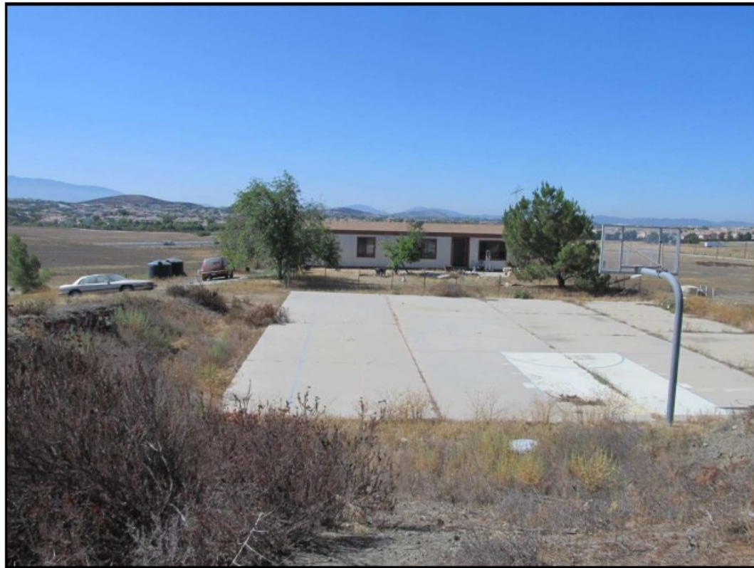
Photo 8. Looking south at the secondary residence and basketball court. (November 2016)
