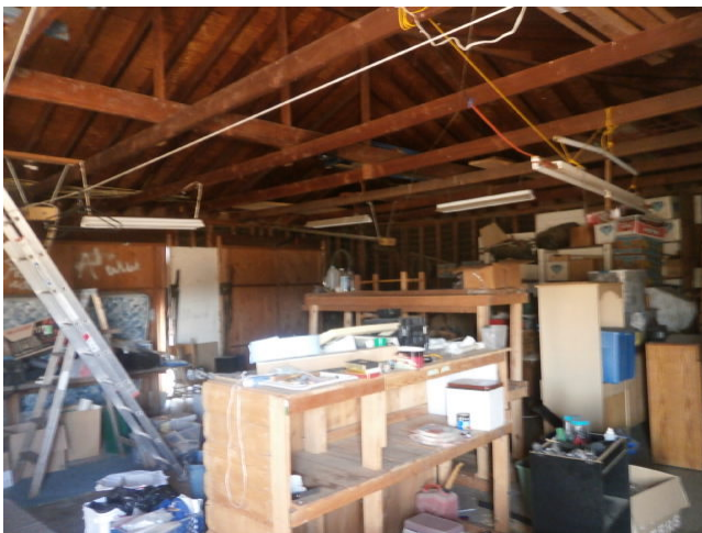
Interior garage structure
