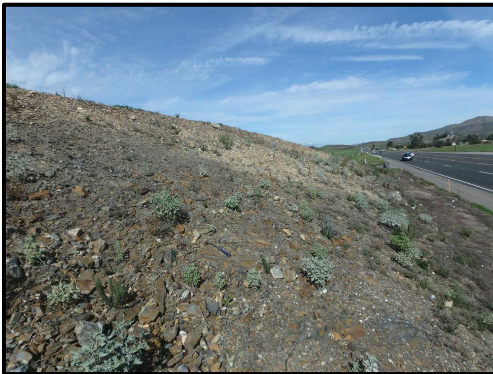
Figure 15. Metamorphic grade bedrock exposed in a rock cut along SR-79 adjacent to the southeastern corner of the survey site. Mapped as Pleistocene-age alluvium (Qvova) and Mesozoic phyllite (Mzp). View northeast.
