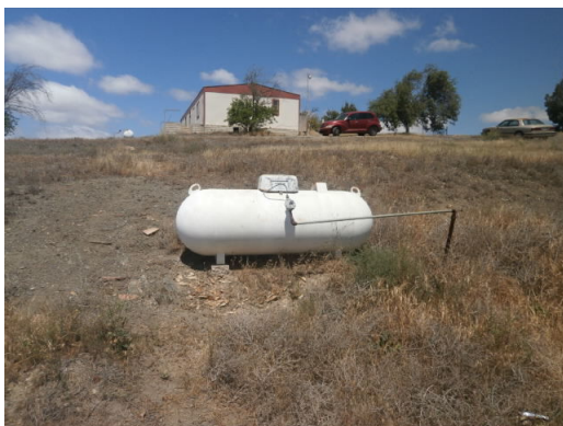
PHOTO #11 PROPANE TANK
