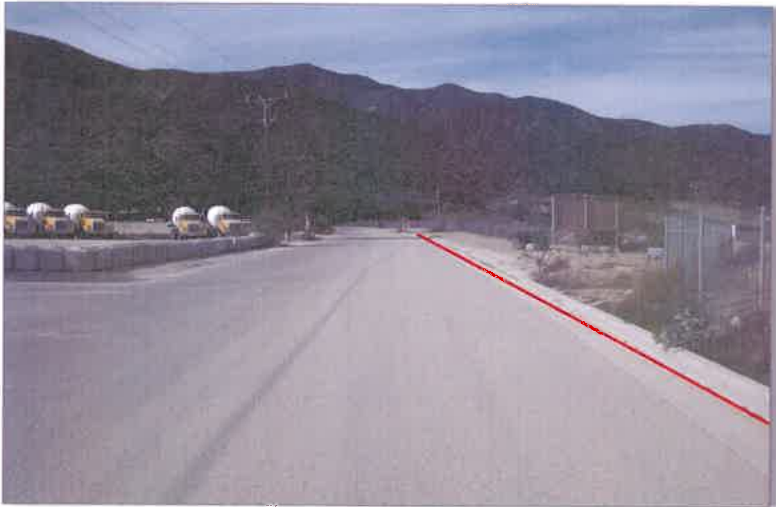
Property line (approximate location shown in red) between SMP143R2 (Left) and SMP 139R1 (Left) (Photograph 4)
