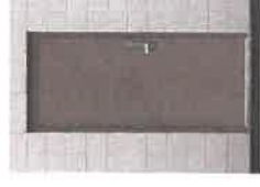
STEEL DOOR (WINE PRODUCTION BUILDING)
