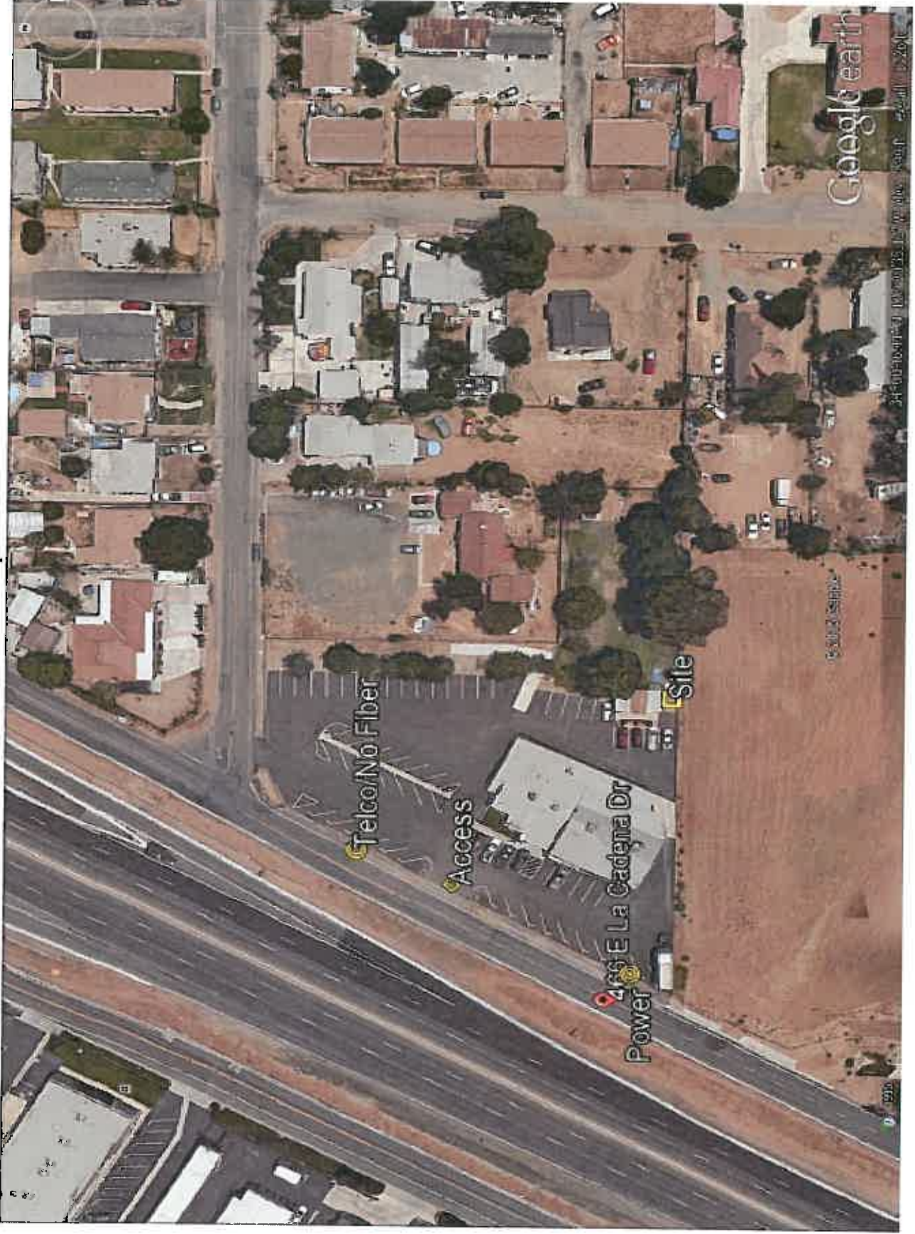
Aerial Photograph of the entire Project Site (Electric)
