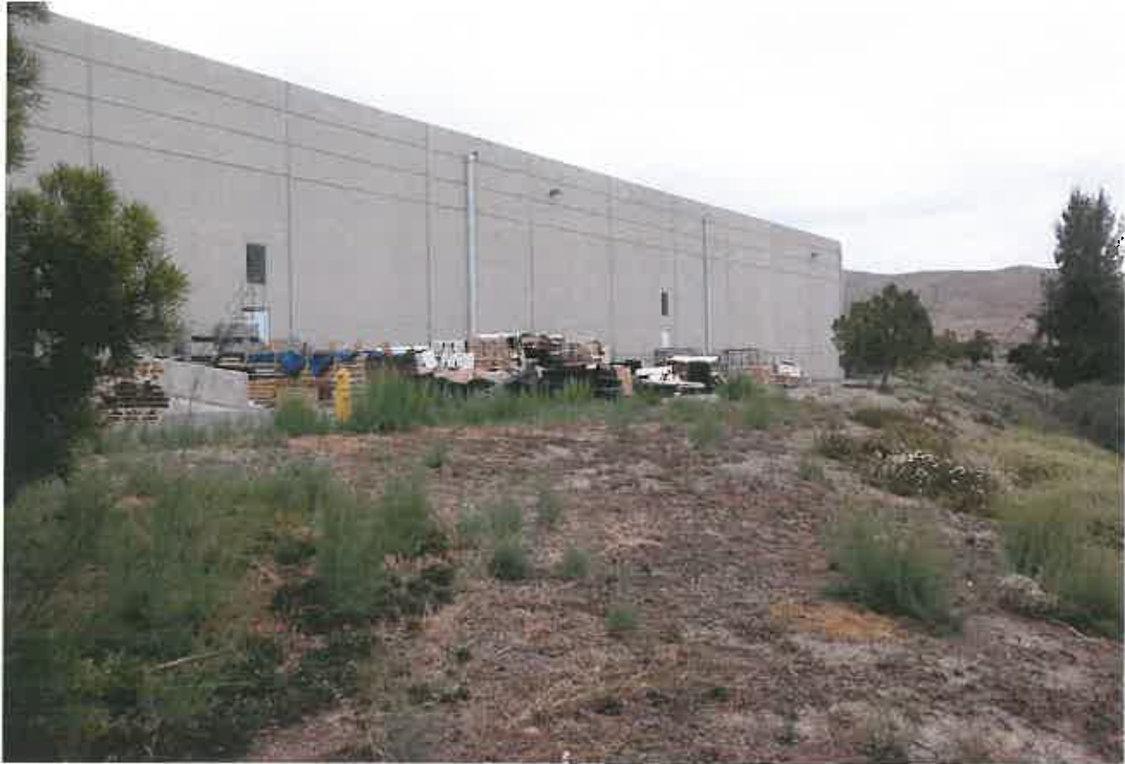
PHOTO # 03: PROJECT AREA #1
