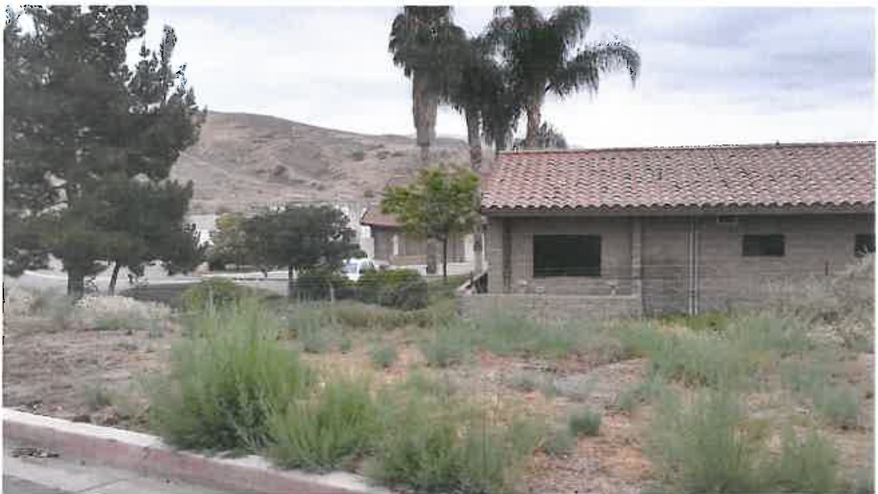
PHOTO # 06: PROJECT AREA #4
