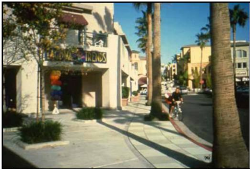
Building design oriented towards the sidewalk
