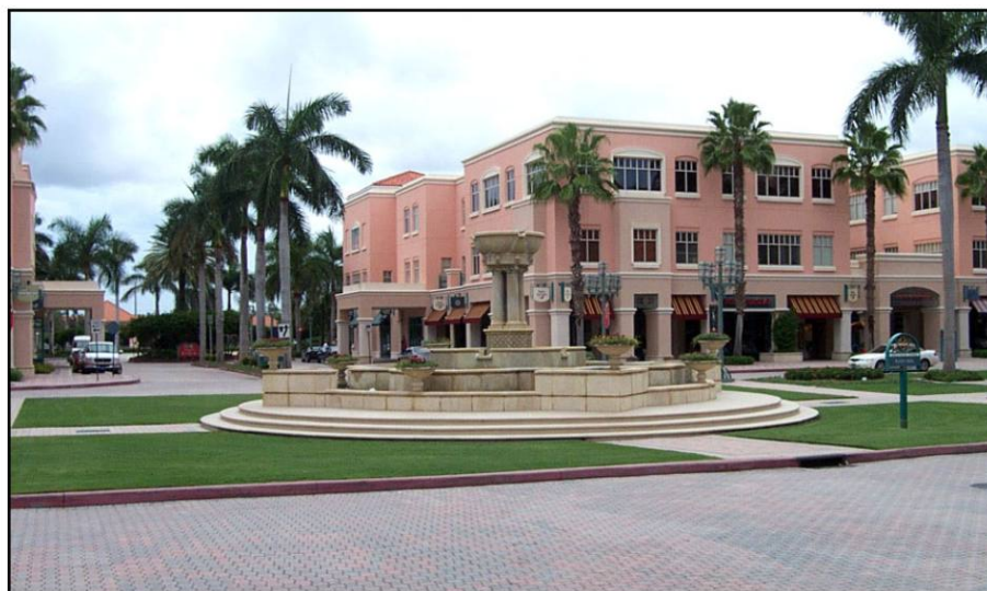
This fountain is a landmark centrally located within this mixed use project.
