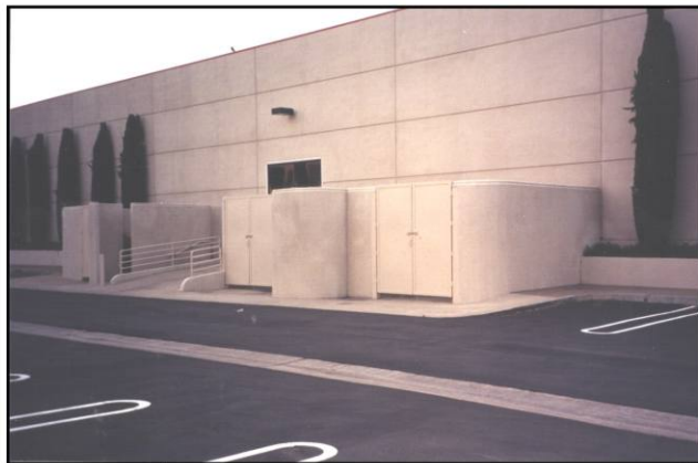
Unightly trash receptacles or mechanical equipment should be screened from view utilizing landscaping or screen walls that compliment the main structure. The enclosures in this photo could be further enhanced by additional landscaping.
