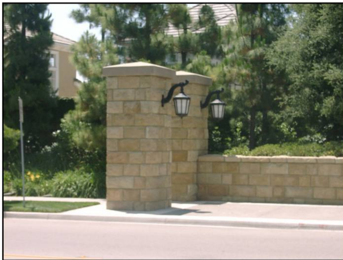
Decorative pedestrian-scale lighting attached to gateway entrance
