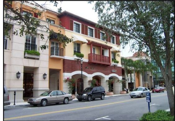
Detailed architectural facade treatment with third story setback, awnings, recessed entryways, arches, and color variety.
