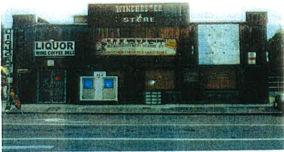
Existing Commercial Building
