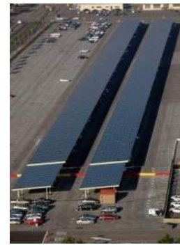
Solar Array at Coronado Naval Base
