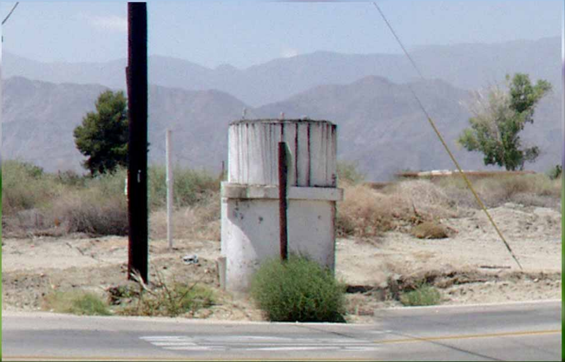
Pressure Regulator Pipes
