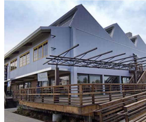
Exhibit 50 | Renovated Packing House
