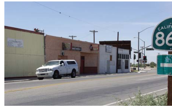
Exhibit 12 | Existing Commercial Buildings
