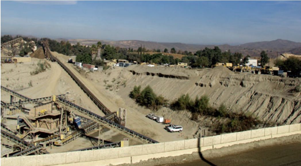
Exhibit 22 | Sand and Aggregate Mining, Temescal Valley
