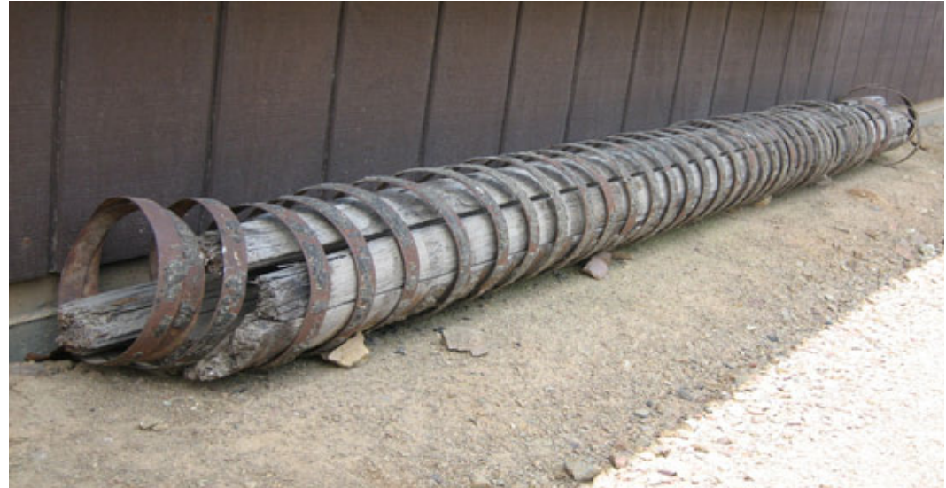
Exhibit 18 | Large Banded Wood Water Pipe
