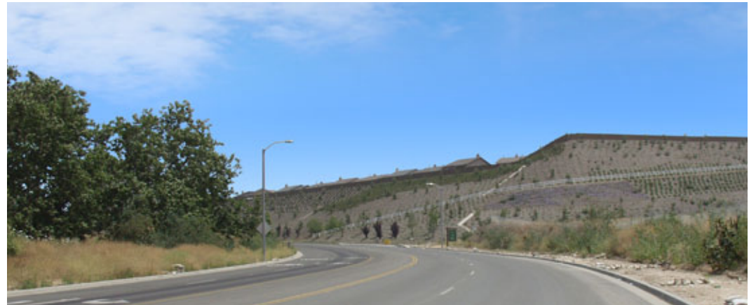
Exhibit 51 | Road C - Campbell/De Palma Road Before Landscape Treatment - Looking South
