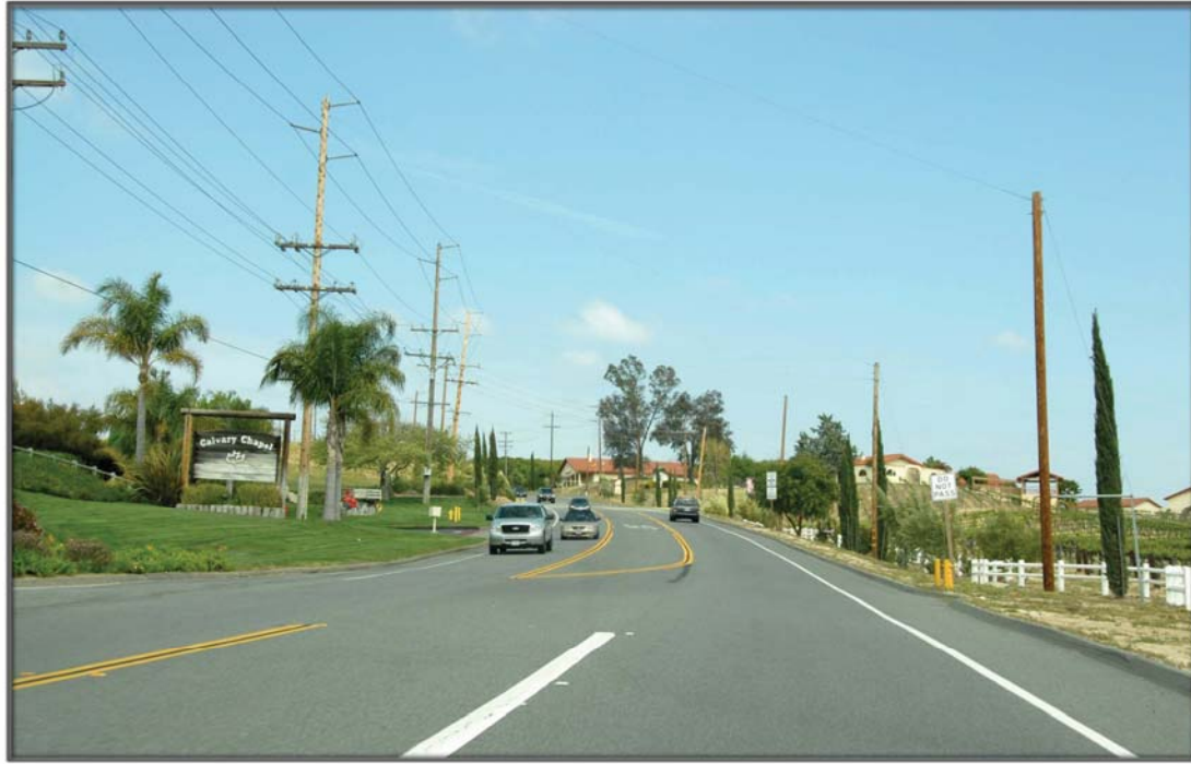
17 Condition 1 – Property Drops Off on Southeast
