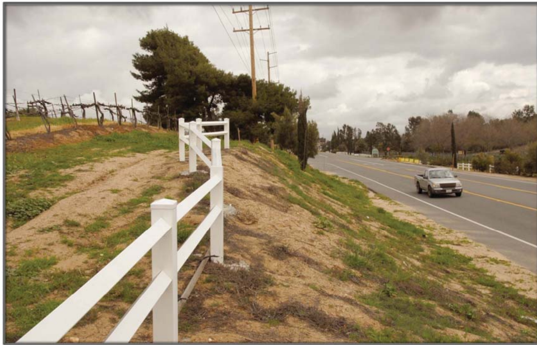
20 Condition #2 – Slope Up on N. Side
