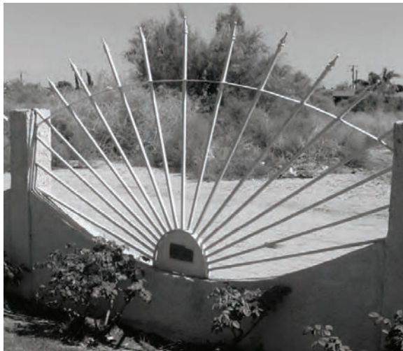
Exhibit 7 | Arch Wall at Catholic Church
