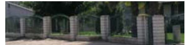
Example of Block and Tubular Steel Fence
