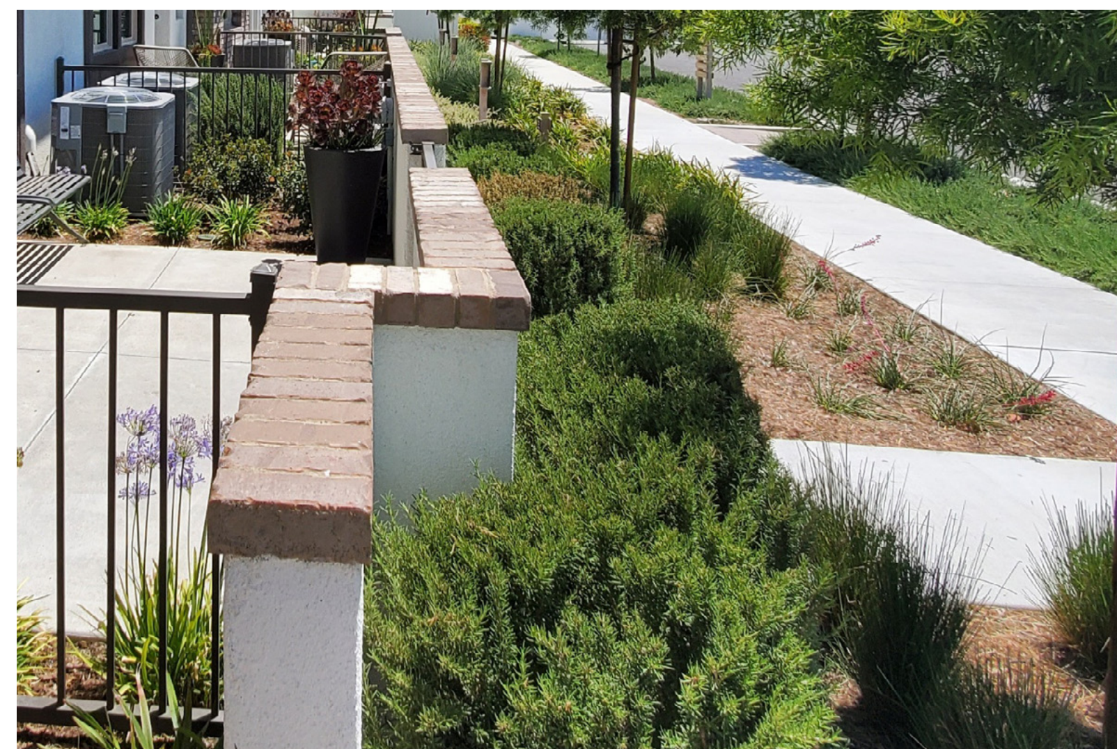
PATIO WALLS Craftsman: Stucco with Brick Cap (color to compliment architecture) Spanish: Stucco with Precast Cap (color to compliment architecture)
