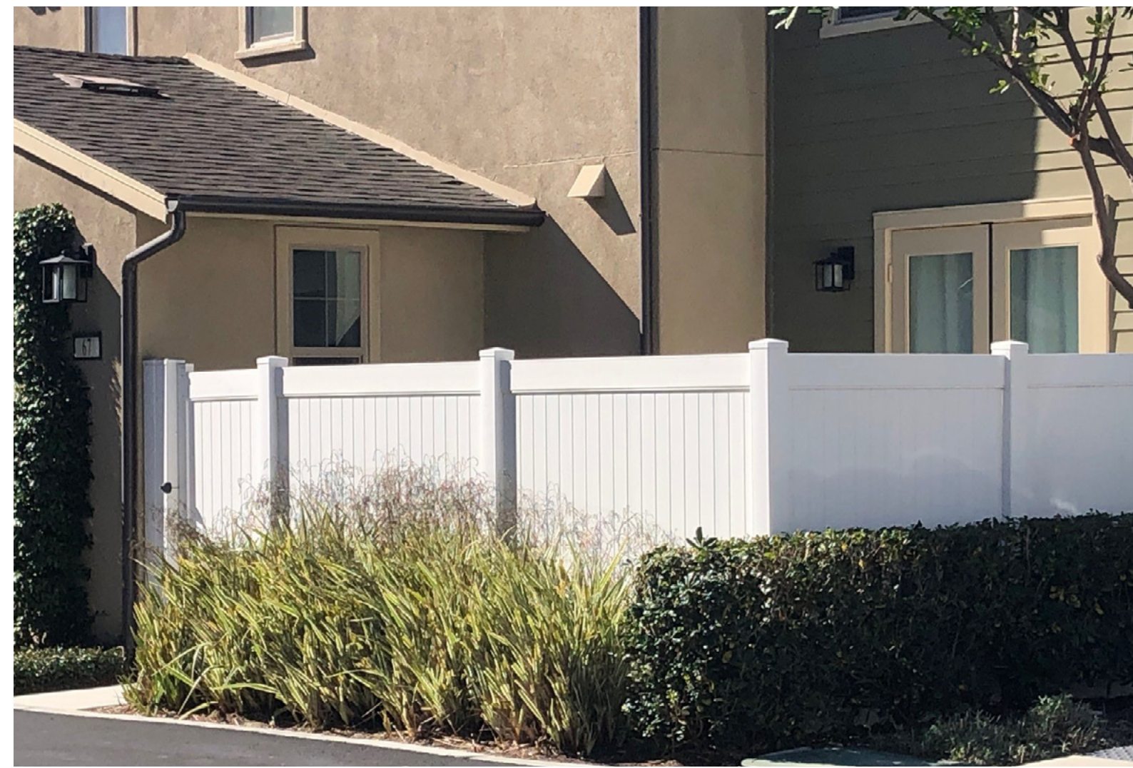
VINYL FENCE (Walls exposed to common areas at end conditions shall be precision block.)
