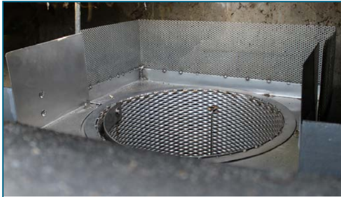
The Curb Inlet Filter features a folding weir that hinges up after the basket is removed to allow easy access to the catch basin if needed.
