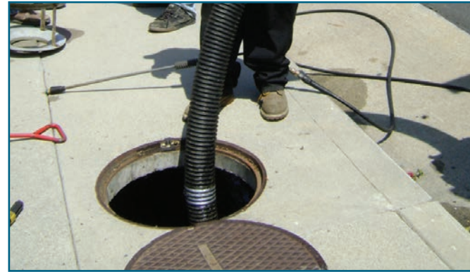
Cleaned easily with vac truck, without catch basin entry, and about 15 minutes is required for service.
