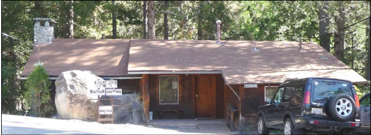
Figure 44: Incorporation of natural features (boulder)
