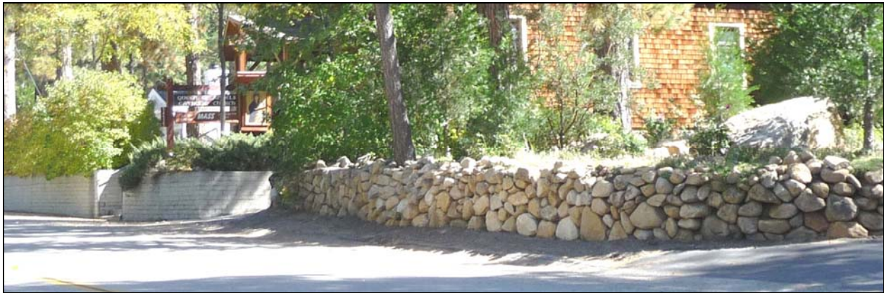
Figure 28: Two types of walls: concrete and rock
