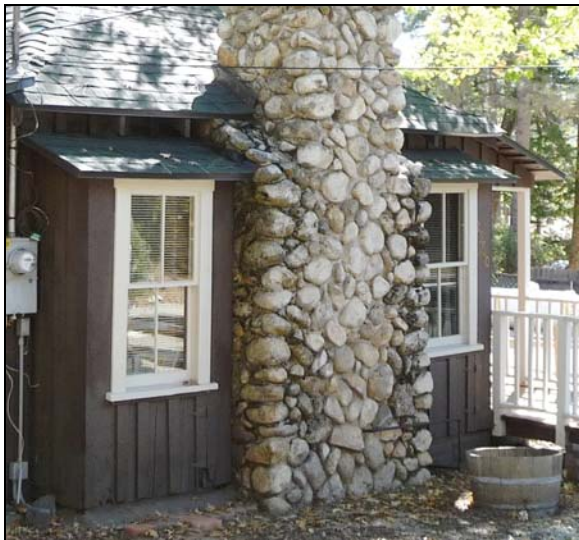
Figure 16: Original, wood-framed double-hung windows with muntins
