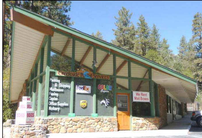
Figure 20: Commercial storefront with fixed windows and wood and glass door.
