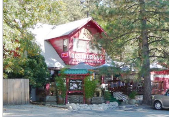
Figure 31: Alterations that have gained historic significance
