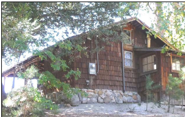
Figure 9: Wood shingle siding
