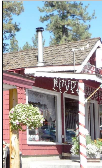
Figure 7: Wood shake shingles
