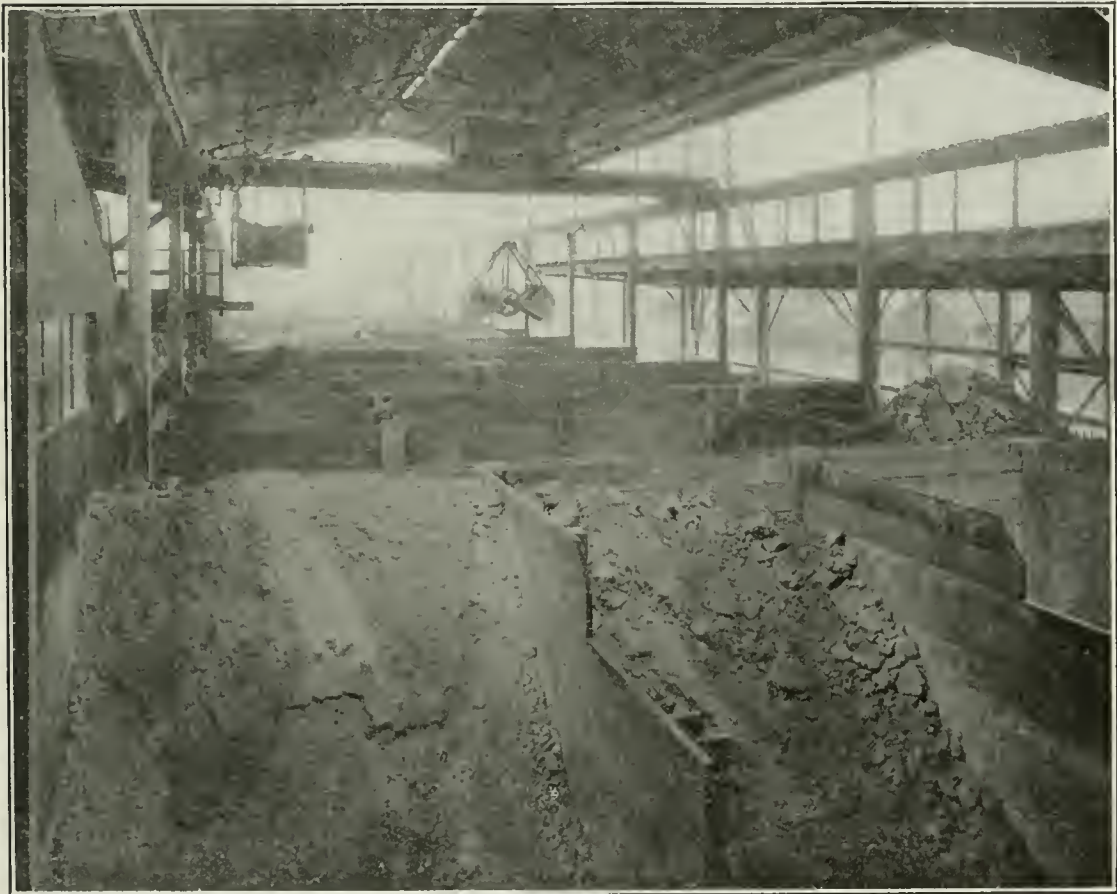
PHOTO No. 20. Clay bins and unloading crane, Lincoln Heights plant, Pacific Clay Products Co., Los Angeles. (Photo by courtesy of the company.)
