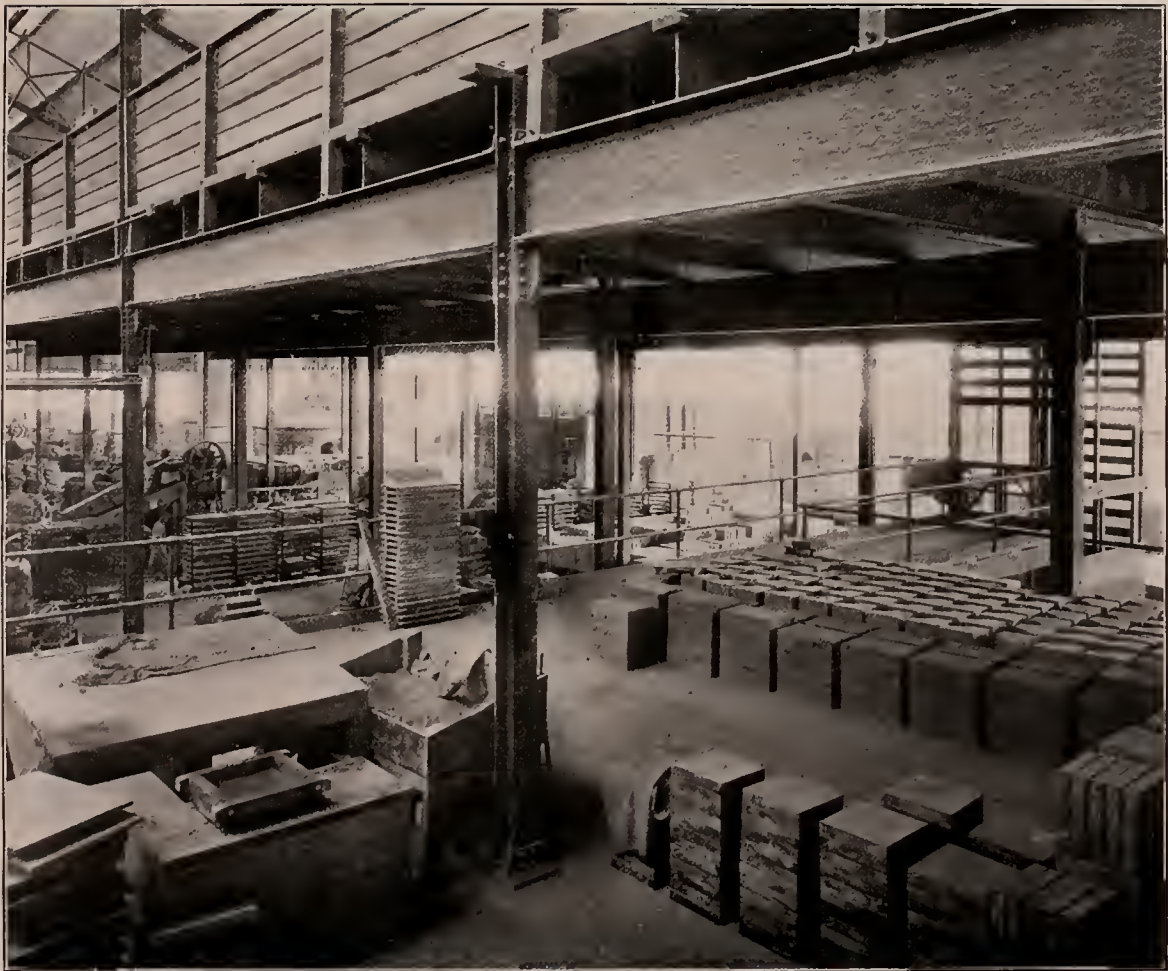
PHOTO No. 24. Interior view of plant, Vitrefrax Company, Los Angeles. (Photo by courtesy of the company.)
