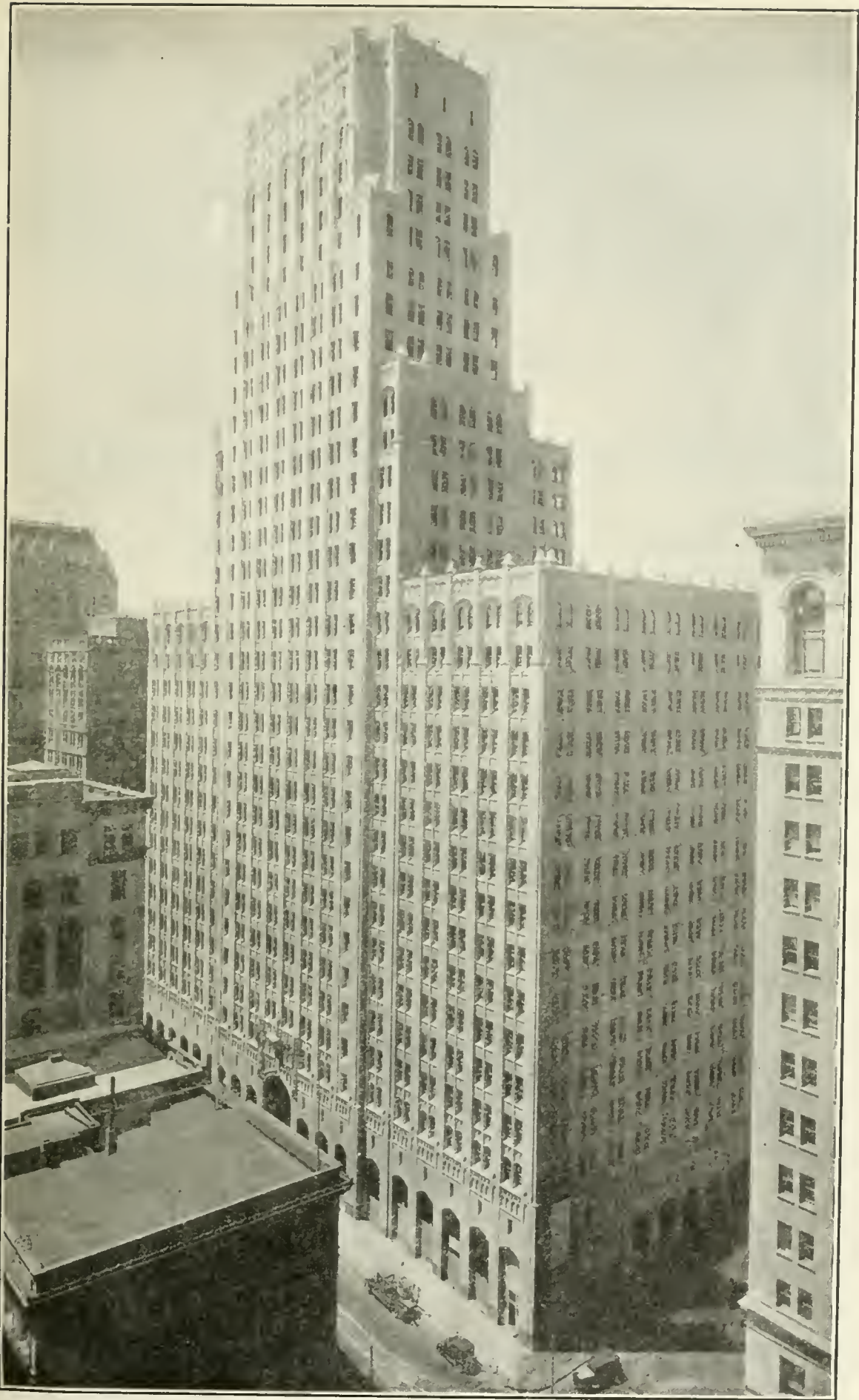
PHOTO No 1, Russ Building, San Francisco, faced with architectural terra cotta manufactured at the Lincoln plant of Gladding, McBean & Co. (Photo supplied through the courtesy of the company.)
