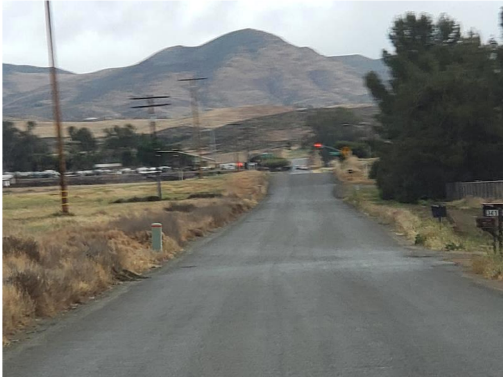
Photo #5 - Looking East Along Old Keller Road. The Project is Located to the Left of the Roadway. This Portion of Keller Road is Scheduled to be Realigned.
