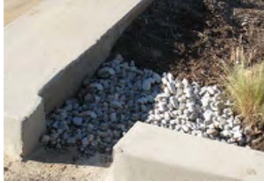
Figure 2: Curb Cut located in a Bioretention Facility
