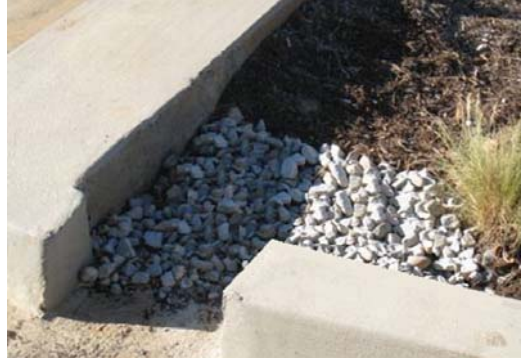
Figure 2: Curb Cut located in a Bioretention Facility
