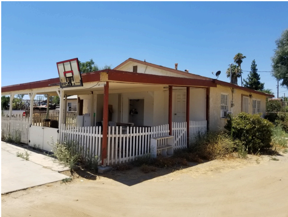
8. East side of the 23085 building
