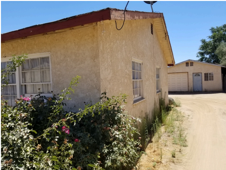
10. West side of the 23085 building
