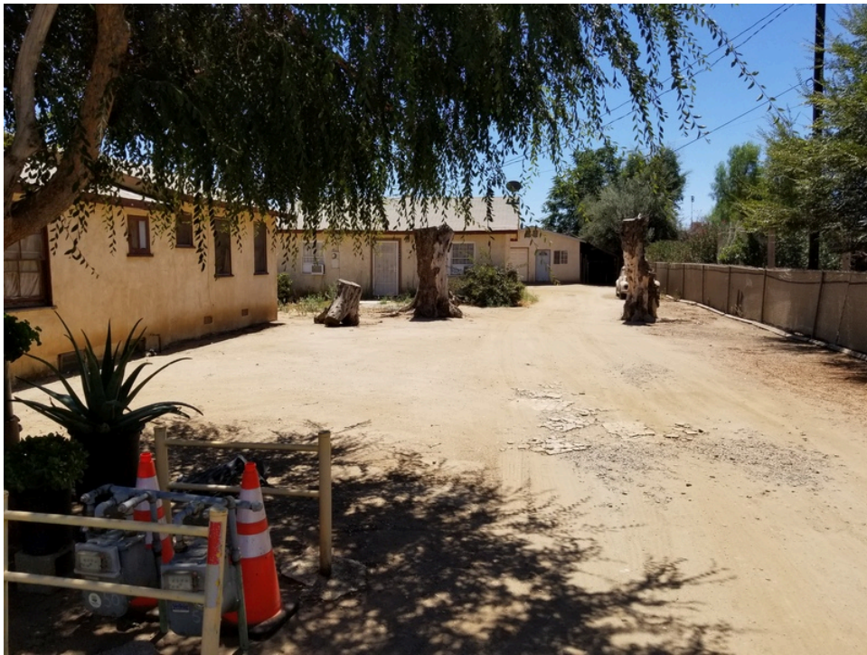
6. Driveway leading to 23085 and garage
