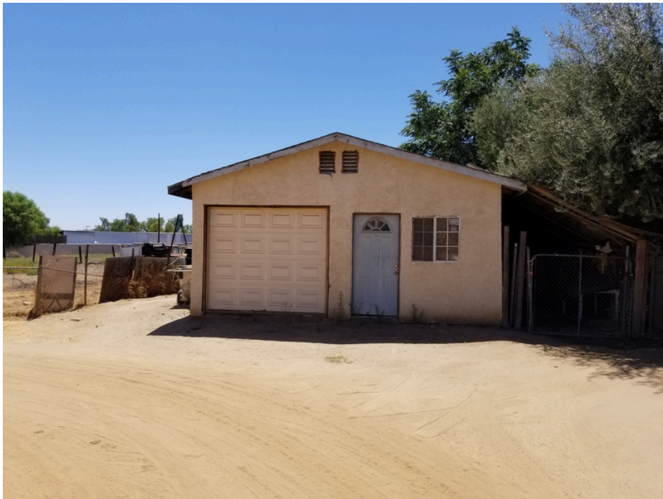
12. North side of subject property garage, facing south
