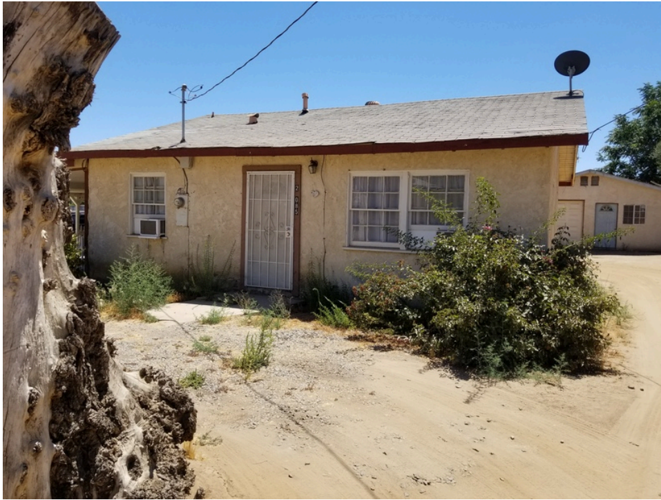
7. North side of the 23085 building
