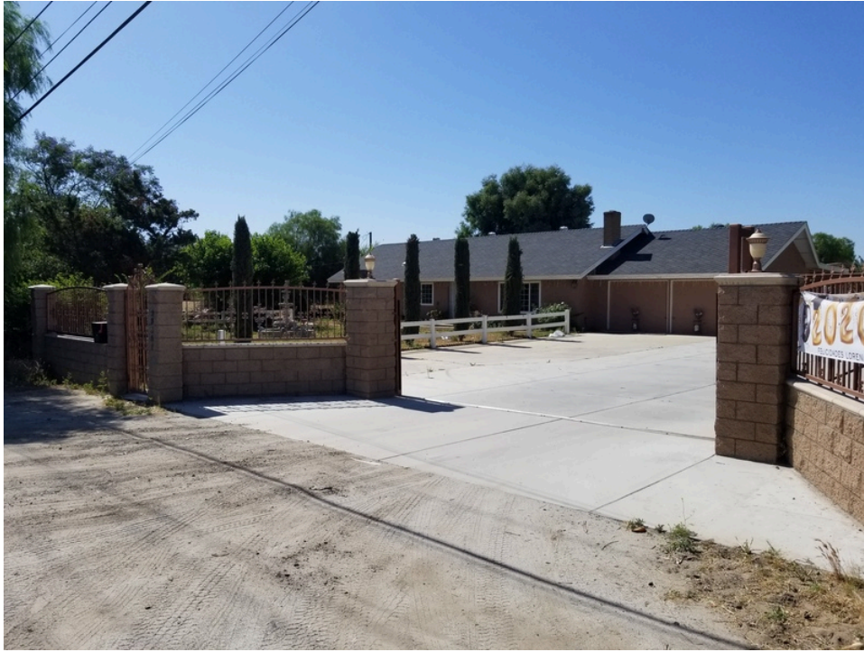
1. Subject property entrance
