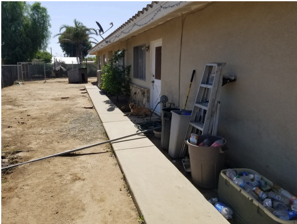
4. North view of subject property building
