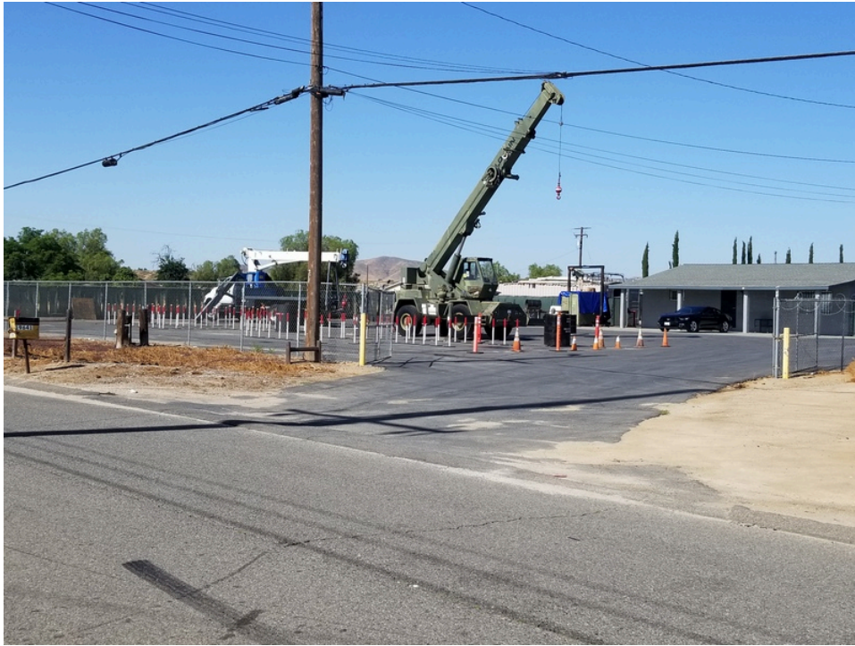
15. West adjoining XL Equipment Sales across Seaton Avenue
