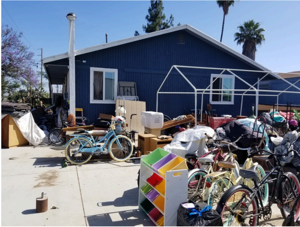
1. Overview of subject property building
