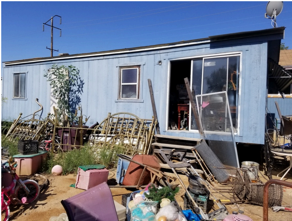
4. East view of subject property building
