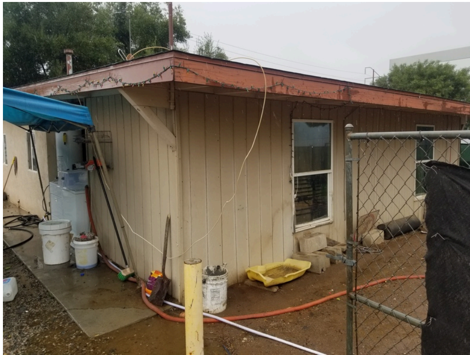
10. Subject property residential building
