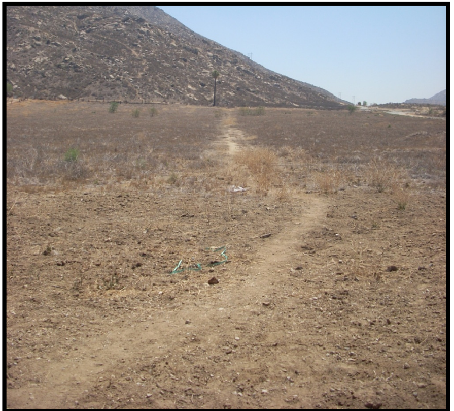
Photo P-10 – Several concrete pipes extending into the subsurface noted along the footpath extending from west to east. Likely associated with a former irrigation system.
