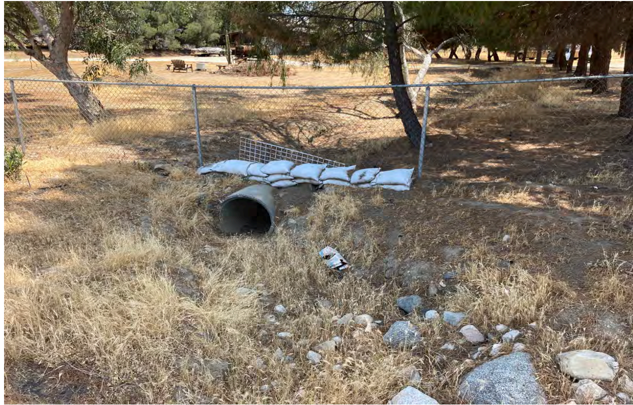
Photograph 21: 02/03/21. View depicting offsite portion of Drainage A looking south.
