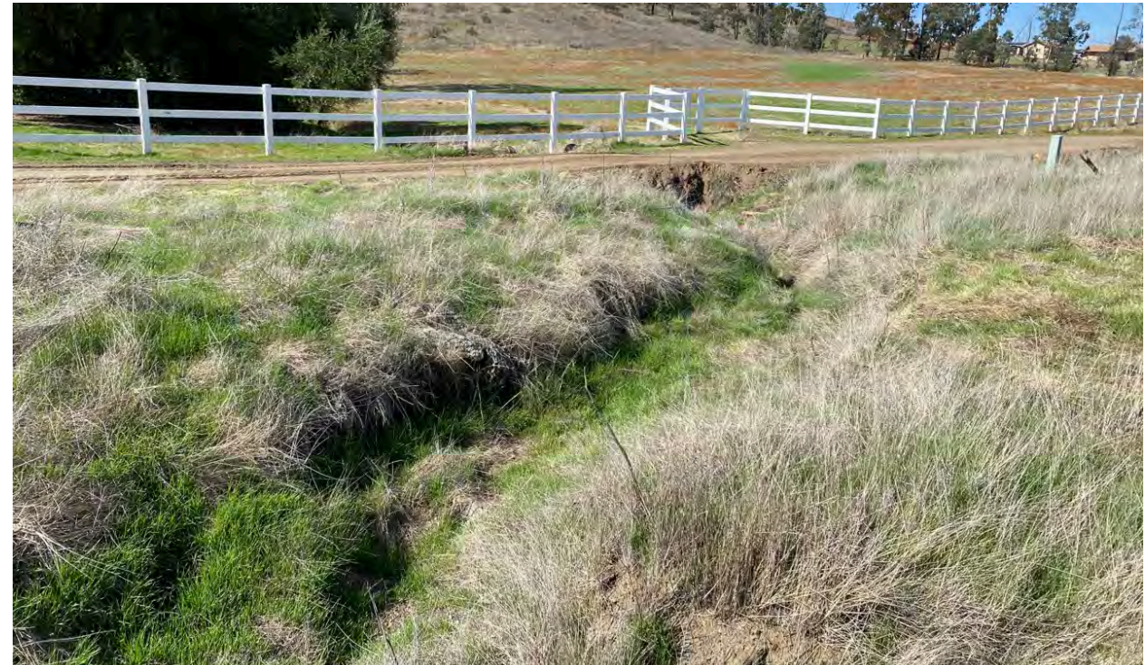
Photograph 4: 02/03/21. Looking at downstream extent of Drainage B towards terminus at culvert.
