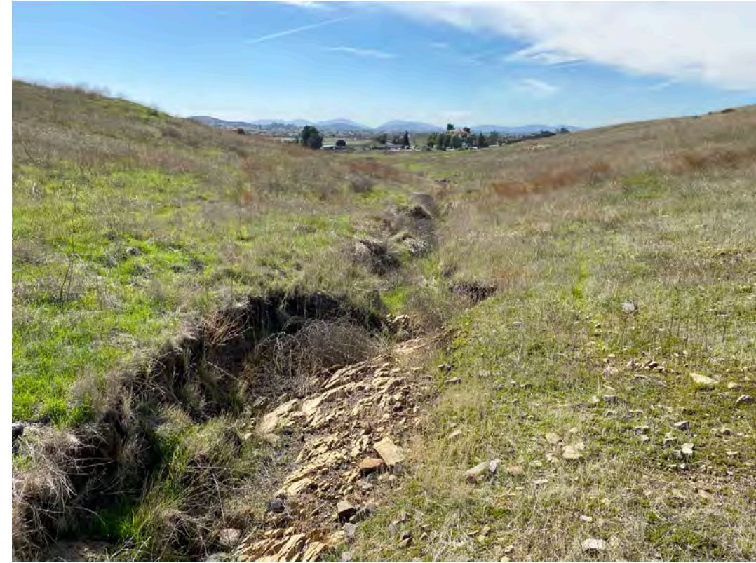
Photograph 10: 02/03/21. Middle portion of Drainage D looking downstream.
