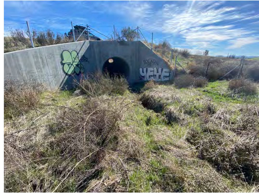
Photograph 18: 02/03/21. Downstream end of Drainage G looking offsite at concrete culvert inlet.
