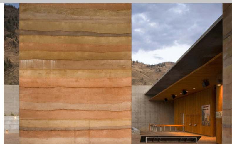
Rammed earth wall
