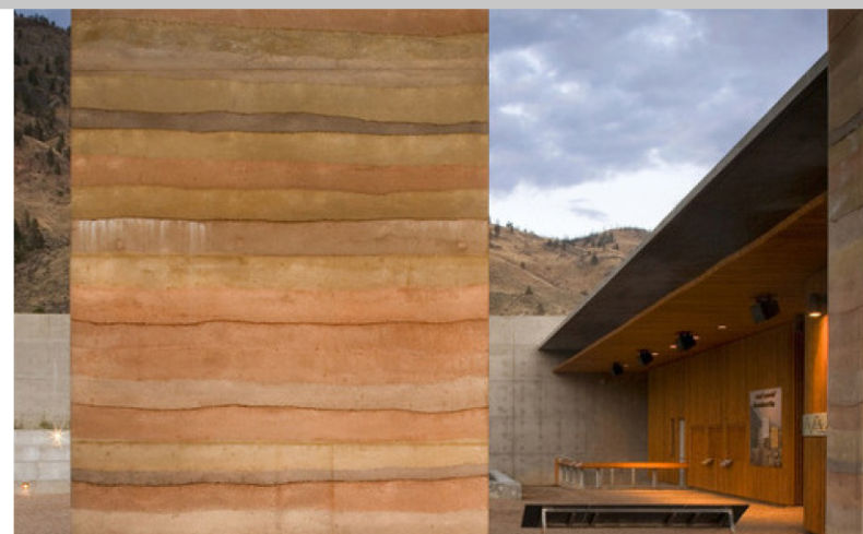
Rammed earth wall
