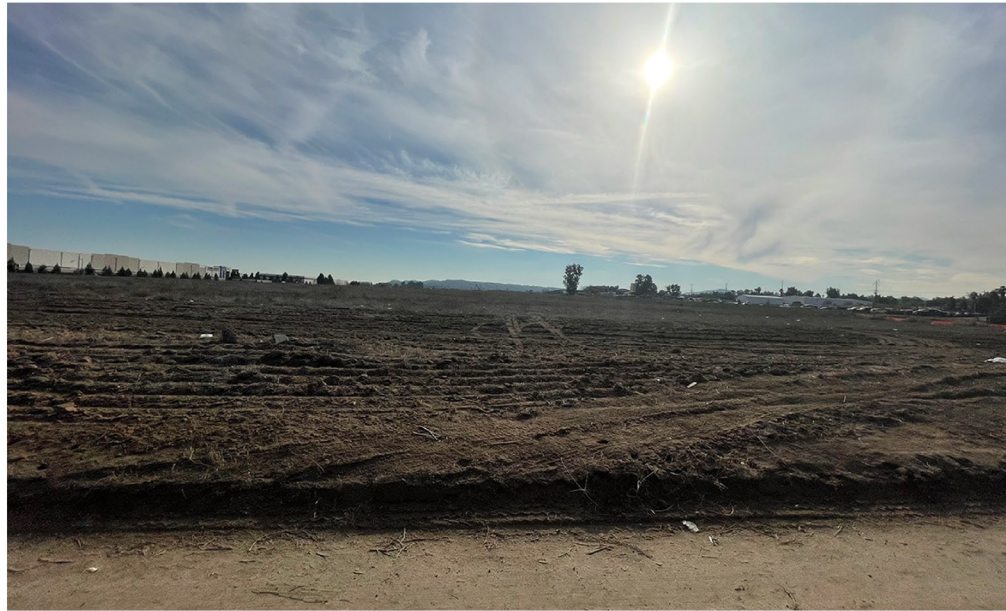
Site Photo 13-1: From northern edge of the project site, along Perry St, facing south.
