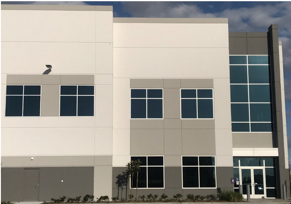
Although provided for illustrative purposes only, the image above shows the repetitive and symmetrical patterns and appropriate styles of windows and doors, desired for buildings in the Stoneridge Commerce Center.
