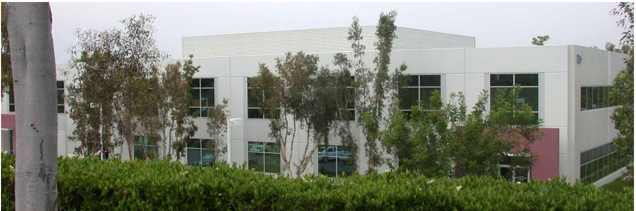
Although provided for illustrative purposes only, the image above shows how rooftop equipment can be screened from public viewing areas.
