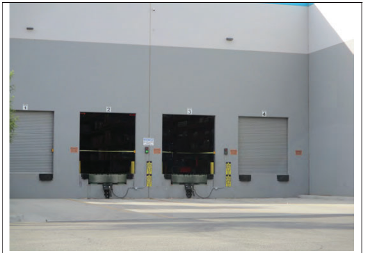
4. View of the loading docks at the Site.
