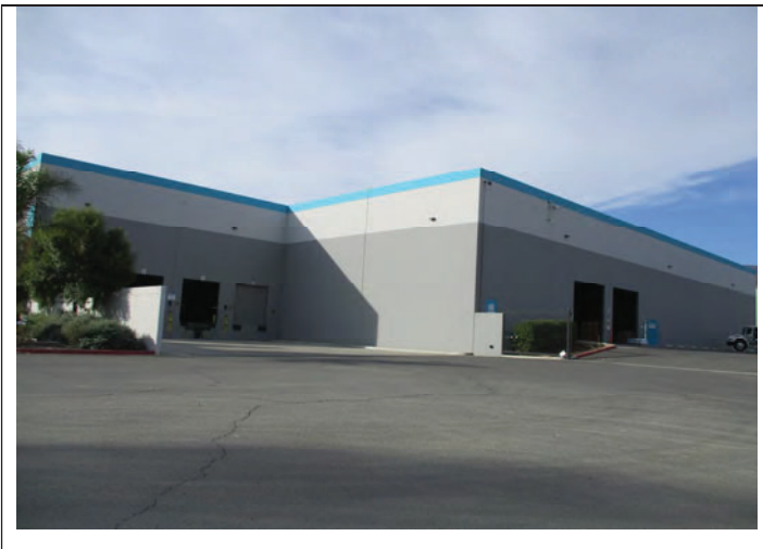
3. View of north side of the Site building.
