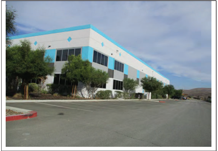
2. View of east side of the Site building.
