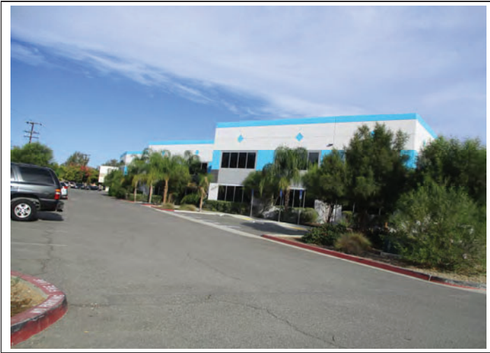
1. View of south portion of the Site building.
