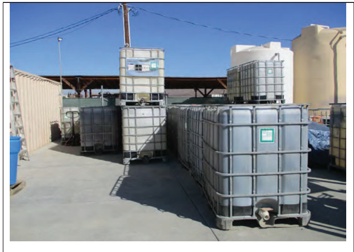
12. View of totes of non-hazardous wastewater at Alpha.
