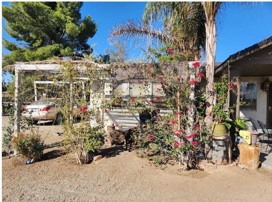
Plate 4.3–27: East façade of the 20111 Patterson Avenue residence, facing west.
