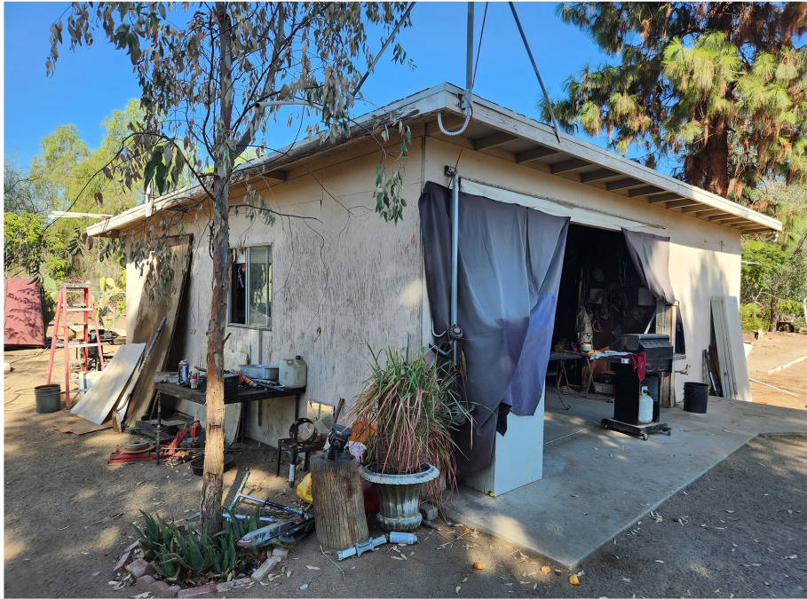
Plate 4.3–40: Southeast corner of the 1977 to 1990 detached garage, facing northwest.
