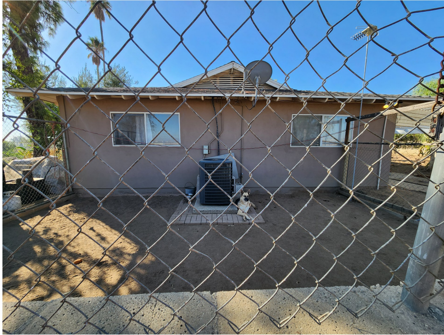
Plate 4.3–19: North façade of the 23330 Walnut Street residence, facing south.
