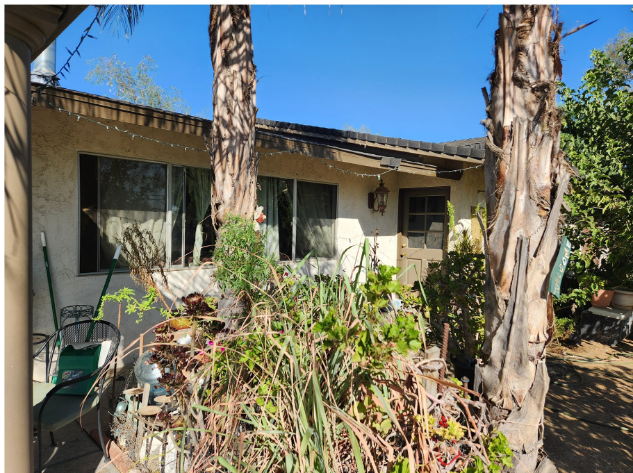
Plate 4.3–28: East façade of the 20111 Patterson Avenue residence, facing northwest.
