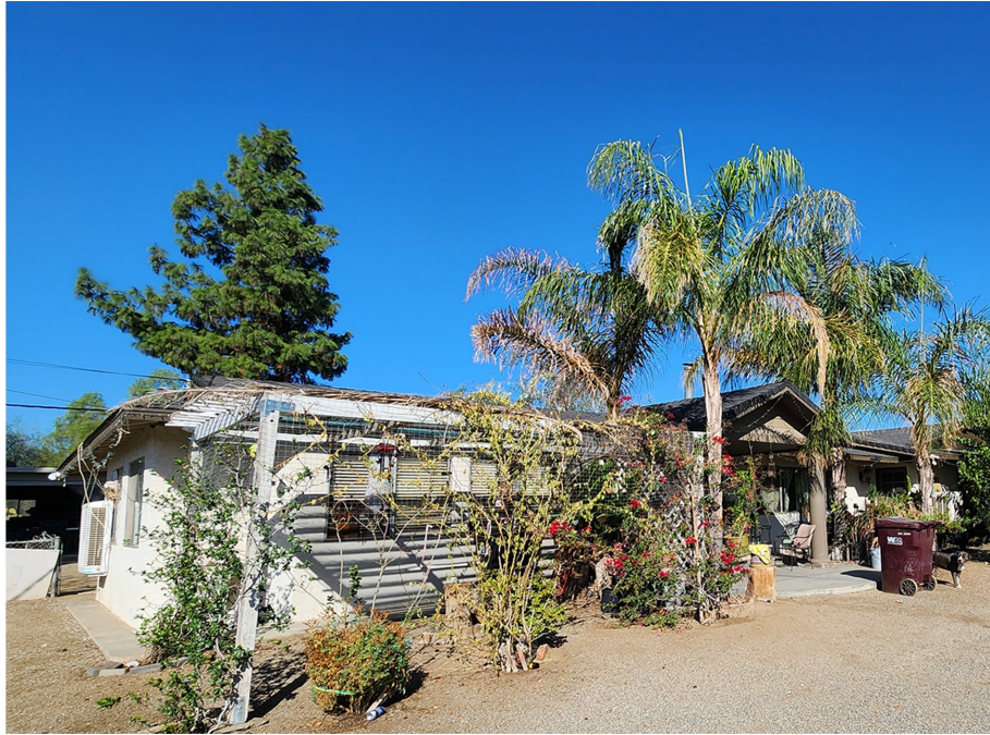
Plate 4.3–25: East façade of the 20111 Patterson Avenue residence, facing northwest.
