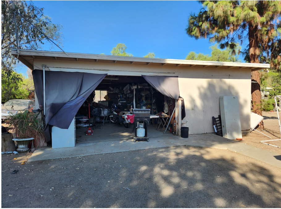
Plate 4.3–39: East façade of the 1977 to 1990 detached garage, facing west.
