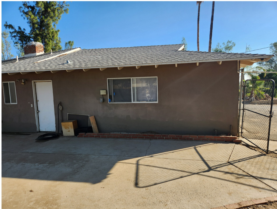
Plate 4.3–14: West façade of the 23330 Walnut Street attached garage, facing east.
