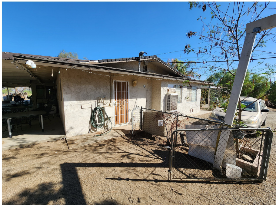
Plate 4.3-35: South façade of the 20111 Patterson Avenue residence, facing northeast.
