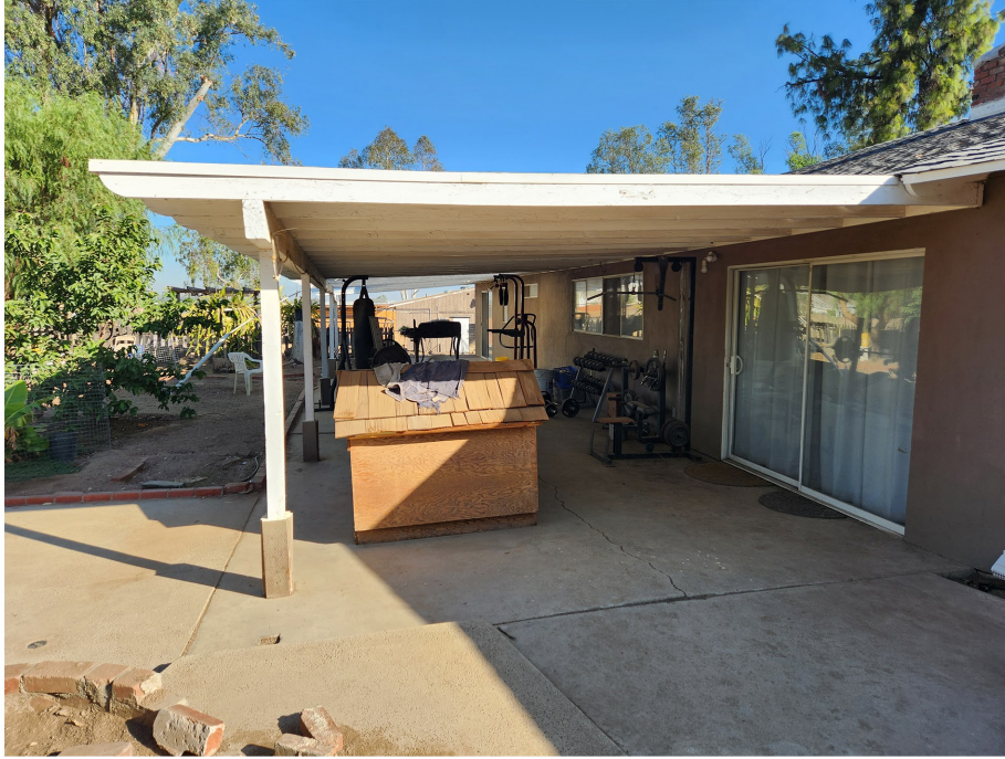
Plate 4.3-15: West façade of the 23330 Walnut Street residence, facing north.
