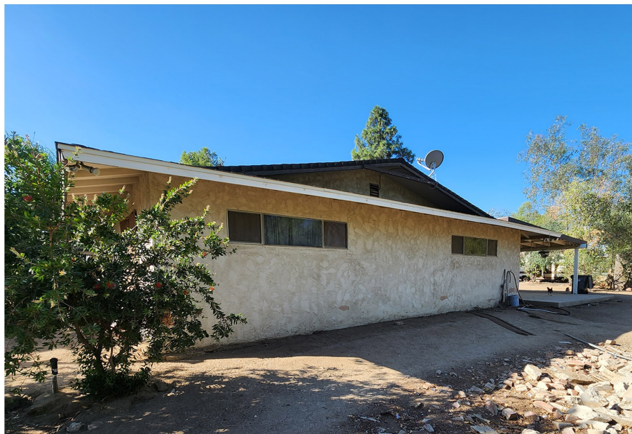
Plate 4.3–34: North façade of the 20111 Patterson Avenue residence, facing southwest.
