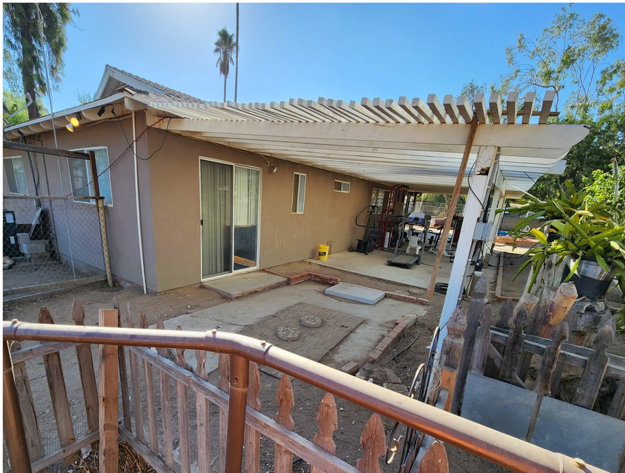
Plate 4.3-16: West façade of the 23330 Walnut Street residence, facing southeast.
