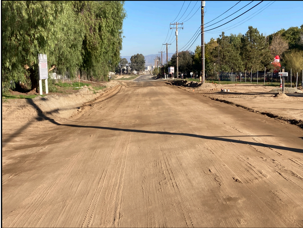
Plate 2: Overview of the intersection of Walnut Street and Patterson Avenue, facing north.
