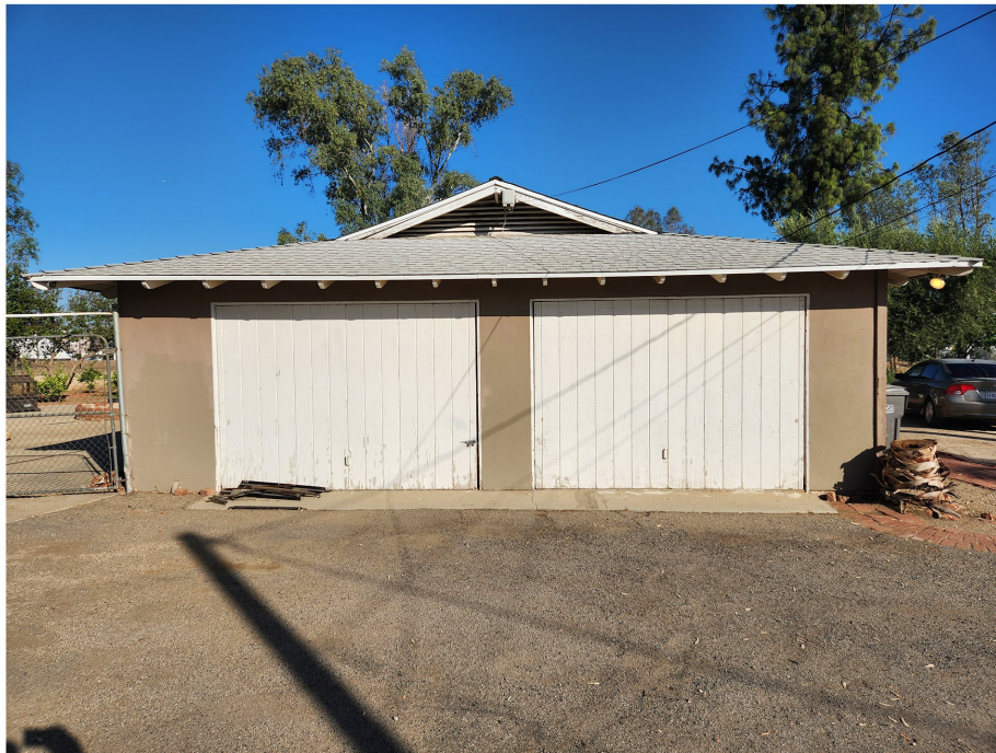
Plate 4.3–20: South façade of the 23330 Walnut Street attached garage, facing north.
