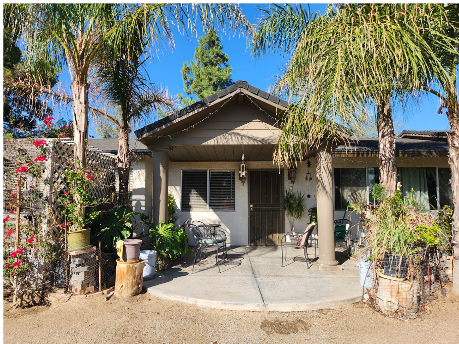
Plate 4.3–26: East façade of the 20111 Patterson Avenue residence, facing west.
