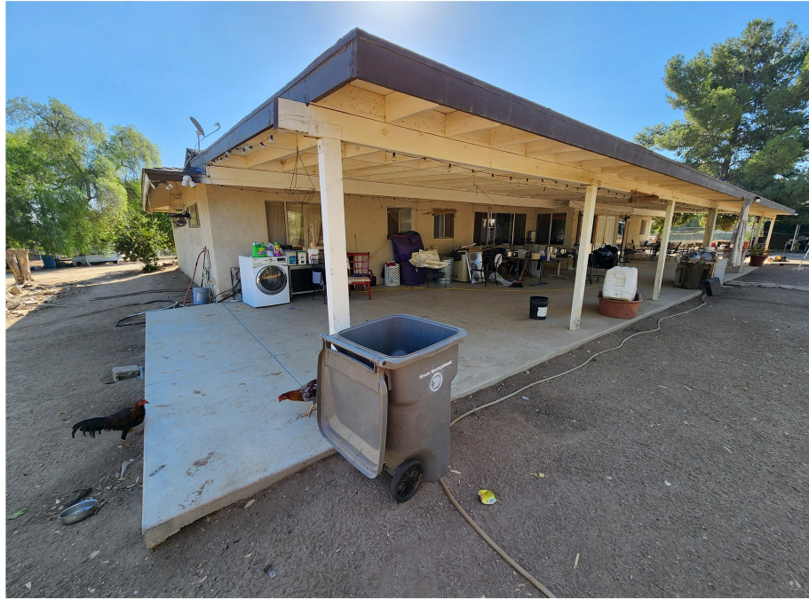
Plate 4.3–29: West façade of the 20111 Patterson Avenue residence, facing southeast.
