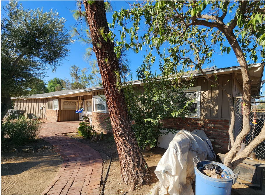
Plate 4.3–8: East façade of the 23330 Walnut Street residence, facing southwest.
