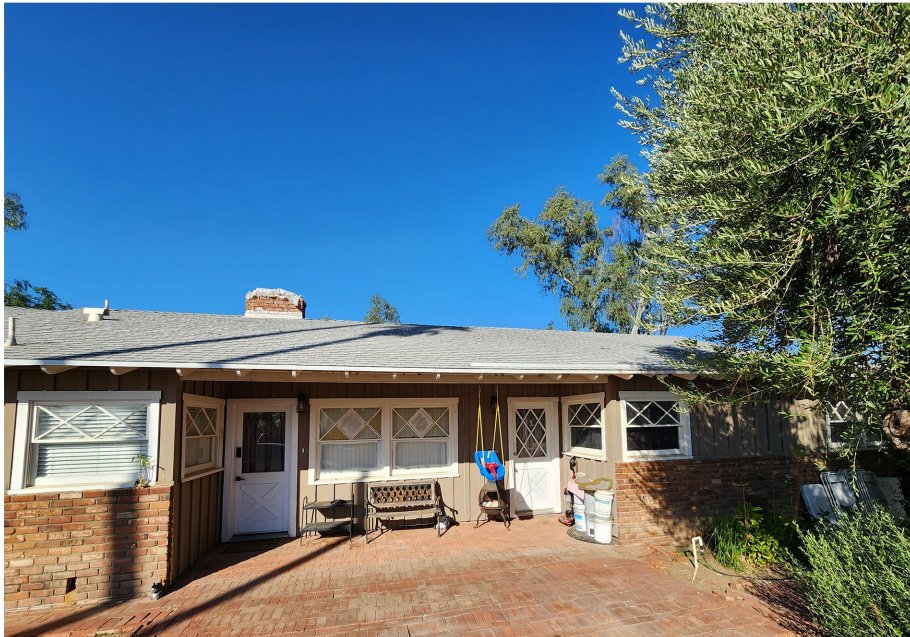
Plate 4.3-10: East façade of the 23330 Walnut Street residence, facing west.
