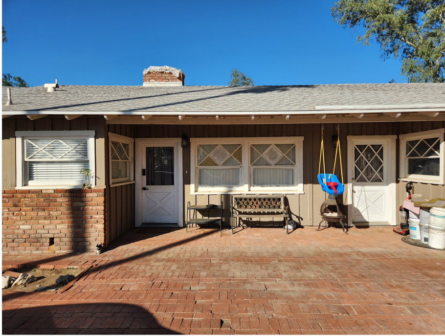
Plate 4.3-9: East façade of the 23330 Walnut Street residence, facing west.
