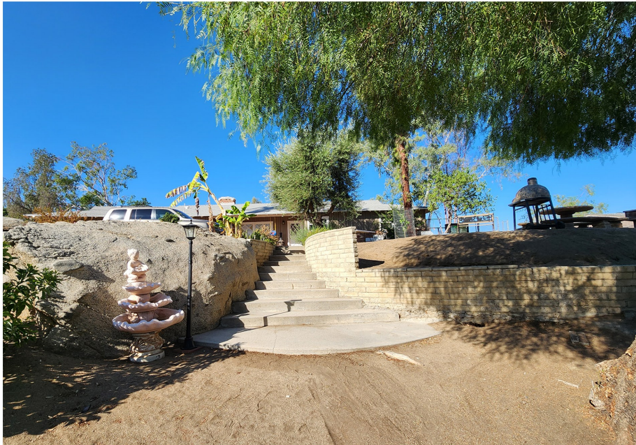
Plate 4.3-6: View of the concrete steps leading to the 23330 Walnut Street entrance, facing west.
