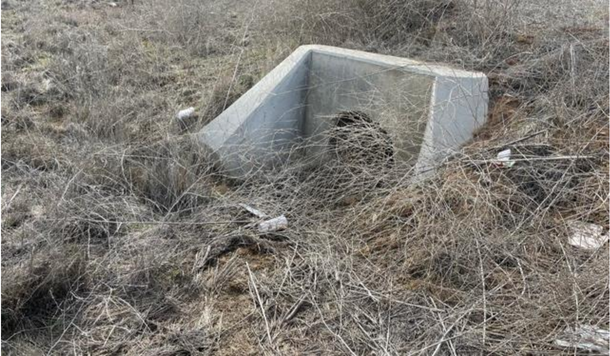
Photograph 1. Culvert entrance under Pourroy Road near the Pat Road intersection.
