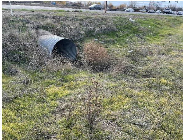
Photograph 6. Existing culverts on the site
