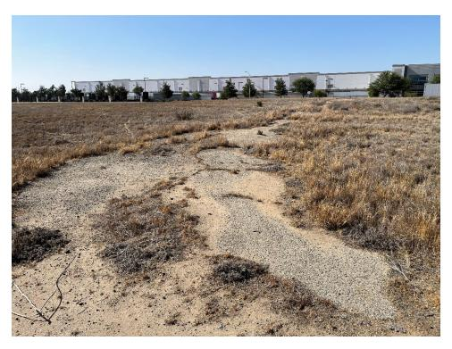
Photo 19 – Remnant of a degraded asphalt driveway on southwestern portion of the Property.
