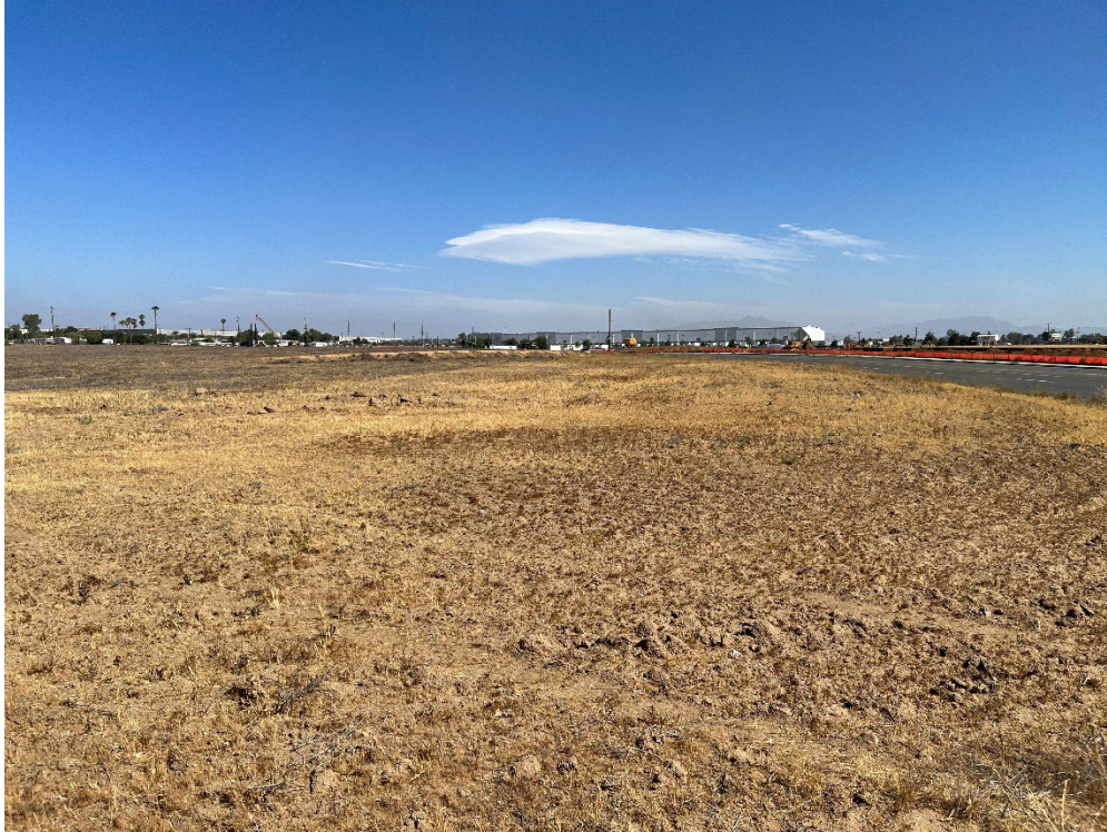
Photo 1 – View from southeastern corner of undeveloped Building 14B site looking north. Harvill Avenue is visible at right.
